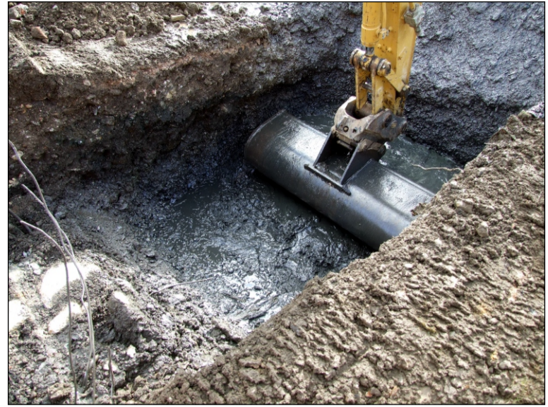
TRENCH 1: FLOODING DURING EXCAVATION
