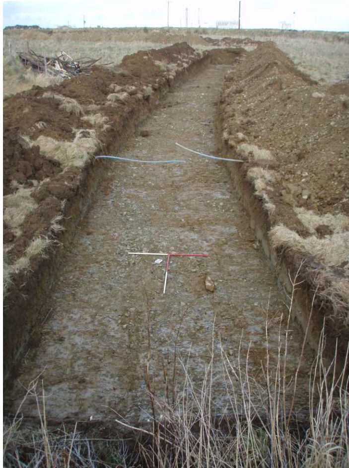
FIGURE 5.1: ENE facing shot of excavated Commercial section footprint Scales 2x1m
