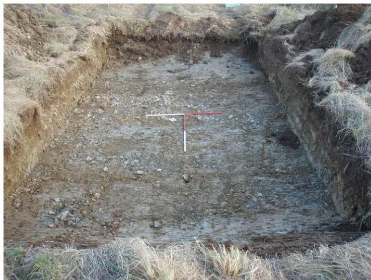
FIGURE 5.2: SE facing shot of excavated Sewage Treatment Plant footprint Scales 2x1m
