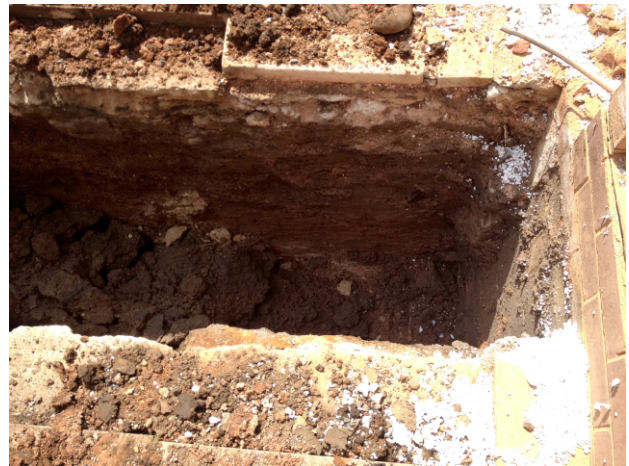
SOUTH FACING SHOT: WEST END OF FOOTING
