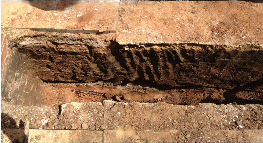
EAST FACING SHOT: NORTHERN END OF FOOTING
