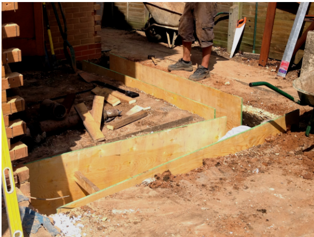
NORTHEAST FACING SHOT: SOUTHEAST CORNER OF FOOTINGS
