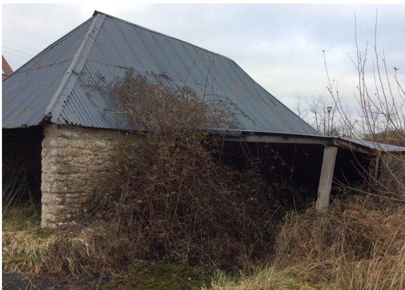
PHOTO 16: LEAN-TO, SOUTH SIDE OF CARTSHED
