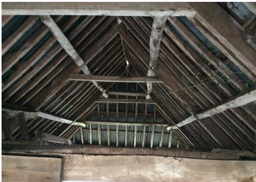
PHOTO 13: CARTSHED, ROOF STRUCTURE, VIEW FROM EAST
