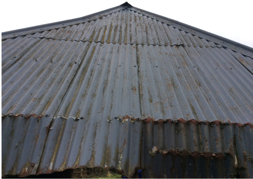
PHOTO 11: CARTSHED, CORRUGATED GALVANISED ROOF FROM EAST END
