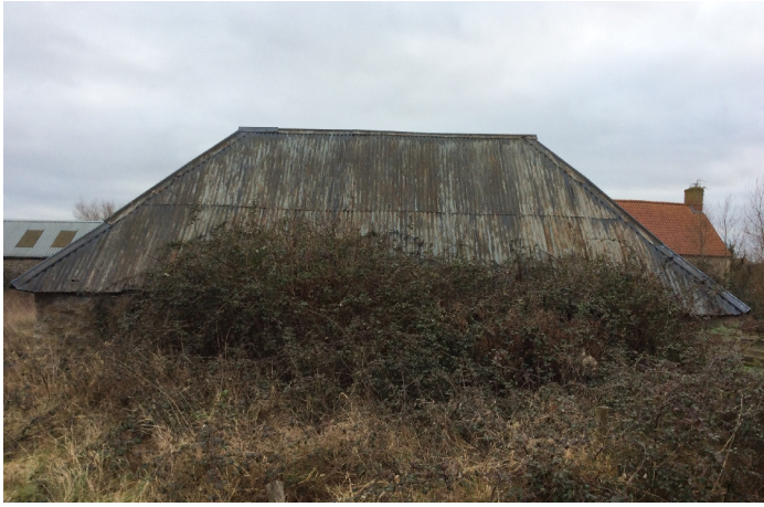
PHOTO 4: CARTSHED, NORTH ELEVATION
