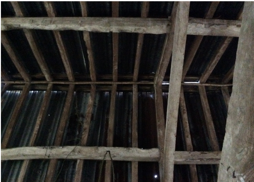
PHOTO 12: CARTSHED, EXPOSED ROOF TIMBERS
