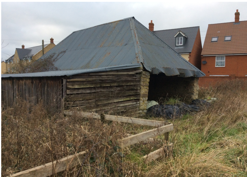
PHOTO 18: LEAN-TO, WEST AND SOUTH ELEVATIONS
