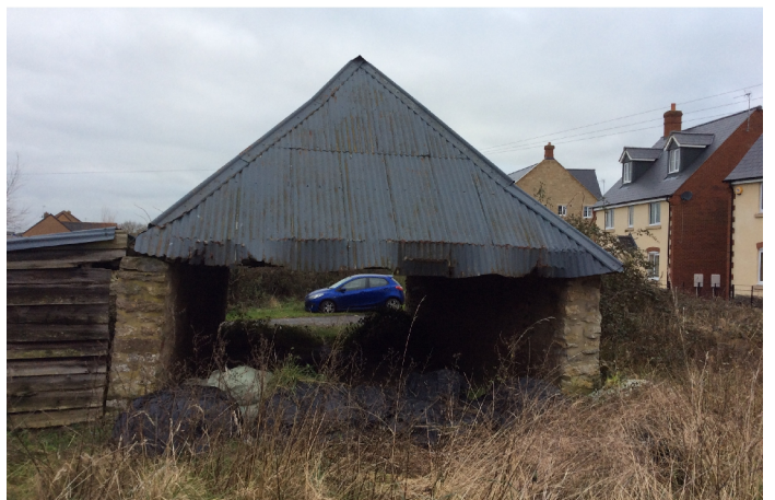
PHOTO 7: CARTSHED, WEST ELEVATION
