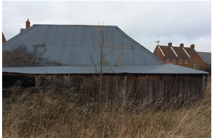
PHOTO 5: CARTSHED, SOUTH ELEVATION
