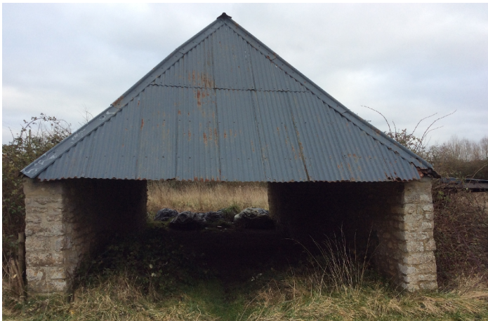
PHOTO 6: CARTSHED, EAST ELEVATION
