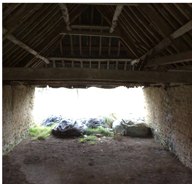
PHOTO 10: CARTSHED, INTERIOR VIEW FROM EAST
