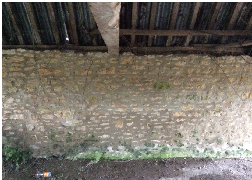
PHOTO 8: CARTSHED, INTERIOR OF NORTH WALL
