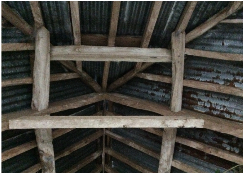
PHOTO 14: CARTSHED, ROOF STRUCTURE, EAST END
