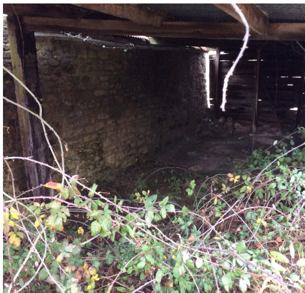
PHOTO 19: LEAN-TO, INTERIOR VIEW
