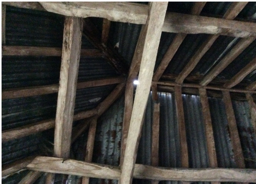
PHOTO 15: CARTSHED, ROOF STRUCTURE, WEST END
