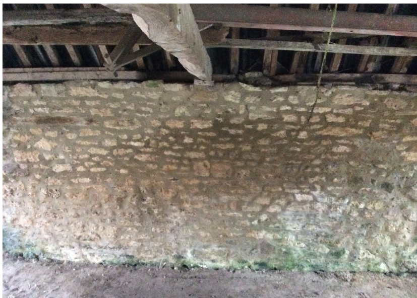
PHOTO 9: CARTSHED, INTERIOR OF SOUTH WALL
