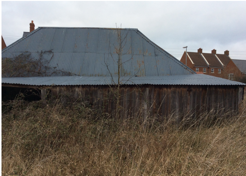
PHOTO 17: LEAN-TO, SOUTH ELEVATION
