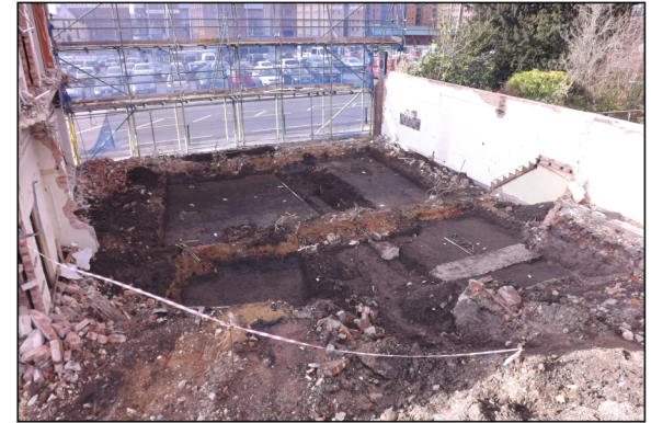
PHOTOGRAPH 6: TRENCHES 3A, B, C and D LOOKING NORTHWEST
