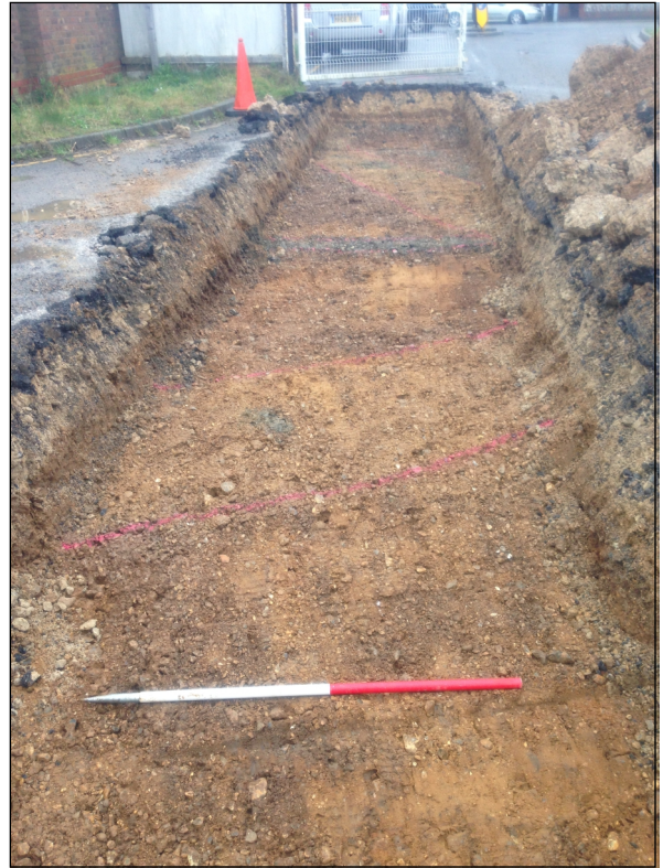
Southern End of Trench 5 looking South
