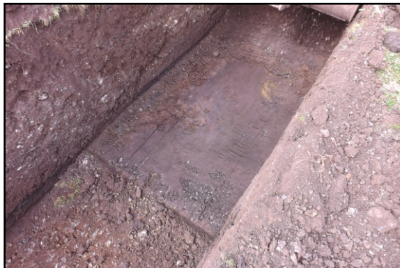
PHOTOGRAPH 5: TRENCH 11 SHOWING BURIED TURF HORIZON (1103) EXPOSED DURING MACHINING
