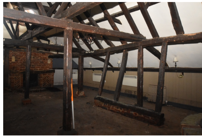
Plate 31: Room I looking to rear
