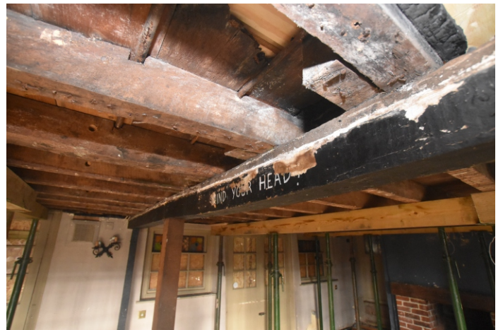
Plate 18: Room D, ceiling beam to right
