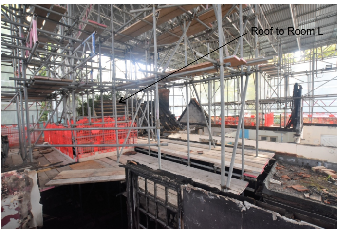
Plate 50: Room L roof
