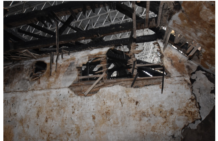
Plate 55: First Floor Room CC looking to rear
