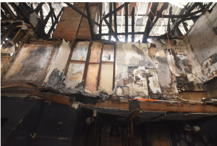
Plate 62: First Floor Room BB, wall to front
