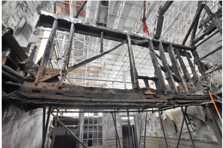
Plate 12: Room C, with rear wall of BB above, beam marking the position of the original rear wall of The Bull
