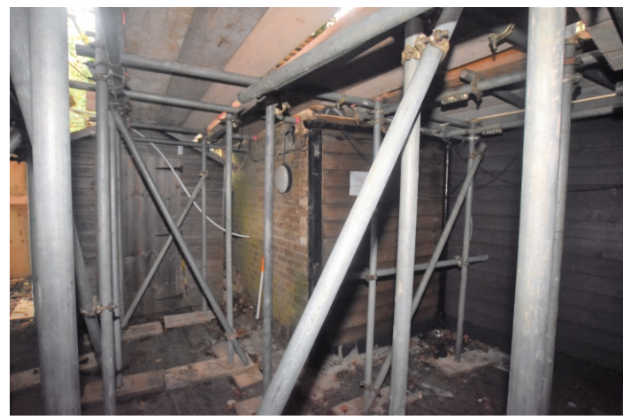
Plate 51: Room L, front right external corner
