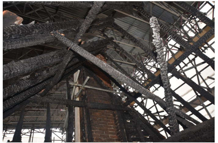
Plate 59: First Floor truss at right gable end
