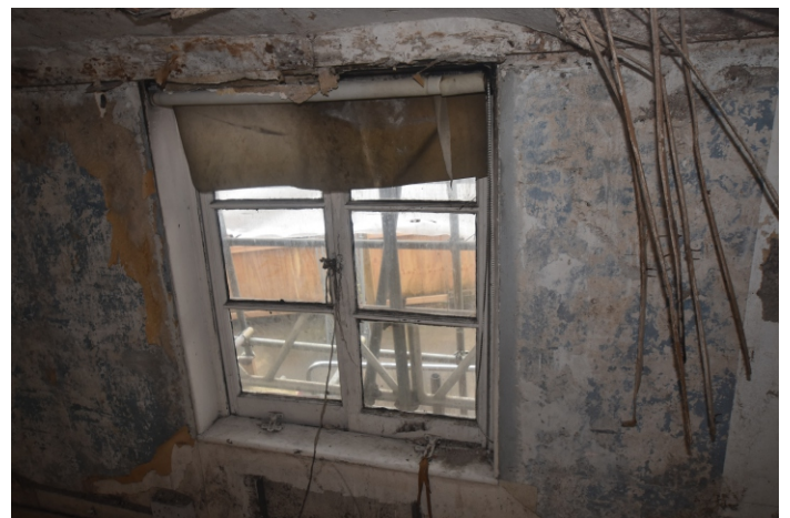
Plate 61: First Floor window detail
