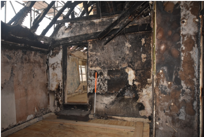
Plate 54: First Floor Room CC looking to left
