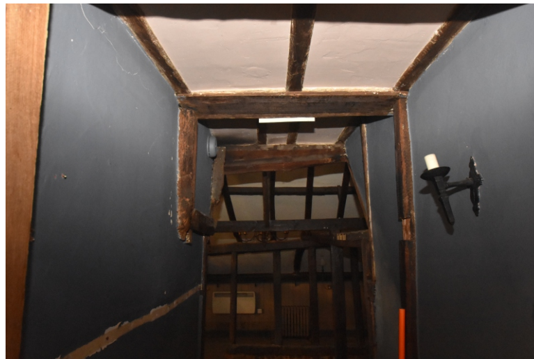
Plate 29: Corridor H looking to right
