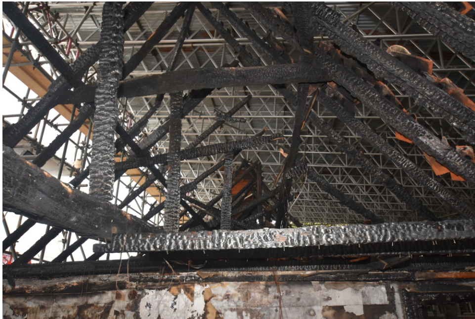
Plate 58: First Floor truss looking left
