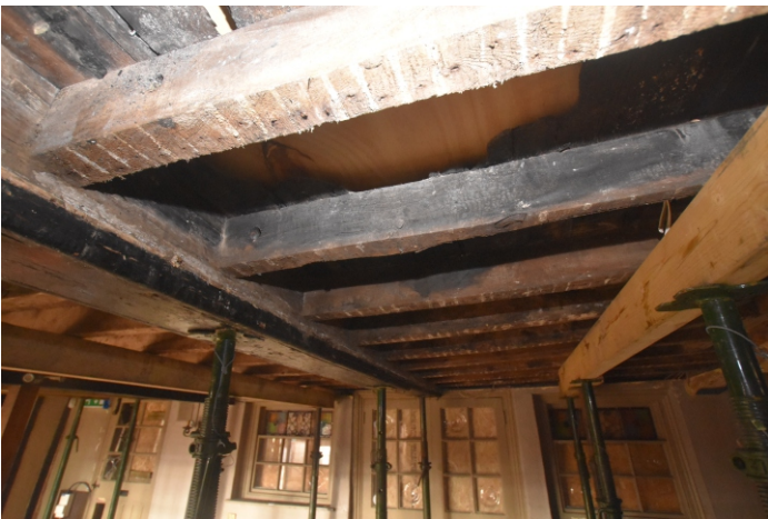
Plate 17: Room D, joists jointed into ceiling beam to left
