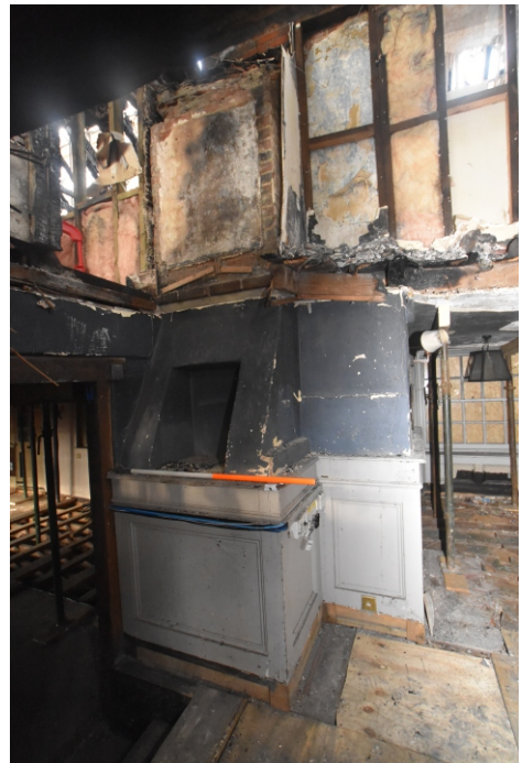
Plate 10: Room B, aperture to rear of chimney stack
