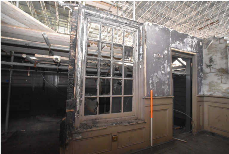
Plate 13: Room C, window and door to rear
