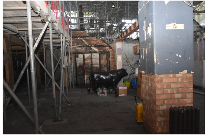
Plate 45: Room J looking to left
