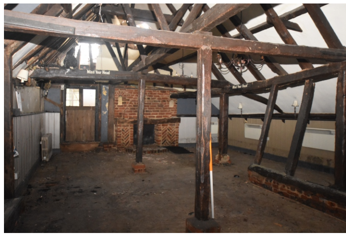
Plate 30: Room I looking to rear
