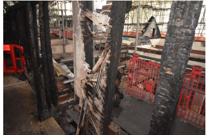
Plate 53: First Floor Corridor AA, lath and plaster
