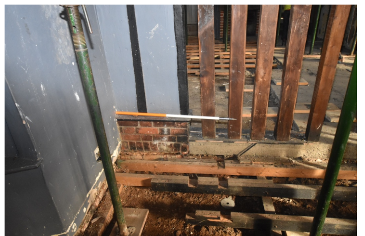
Plate 20: Partition between Rooms D and E, as seen from Room E
