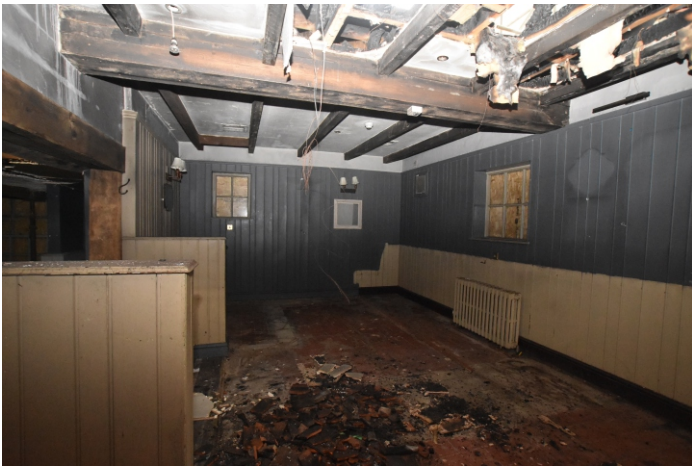
Plate 4: Room A looking to front
