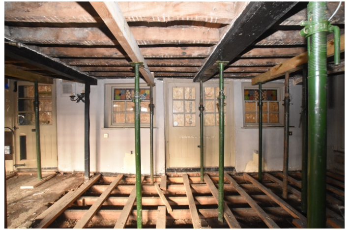
Plate 16: Room D, wall to front showing ceiling beams and doors/windows
