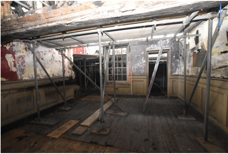
Plate 11: Room C looking to rear
