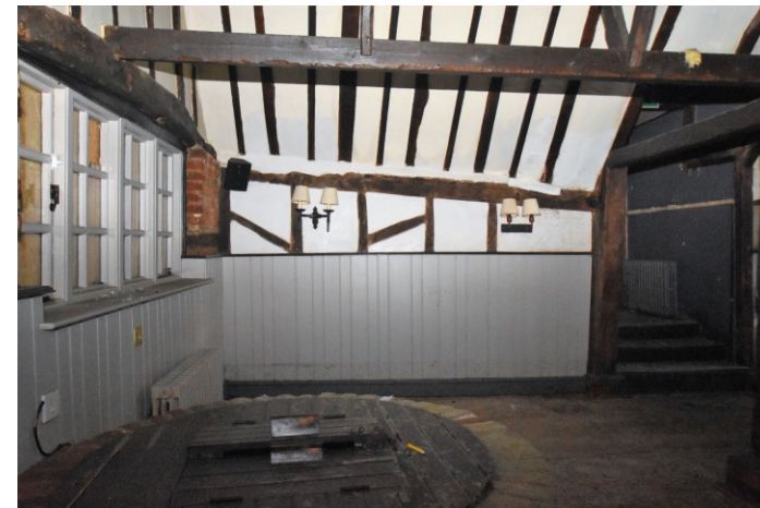
Plate 40: Room I wall to front left
