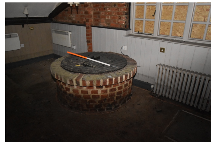
Plate 44: Room I, well to front
