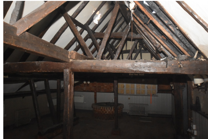
Plate 35: Room I spine beams
