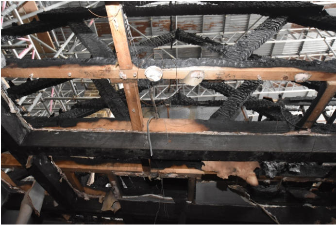
Plate 6: Room A truss
