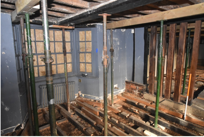
Plate 21: Room E, central ceiling beam
