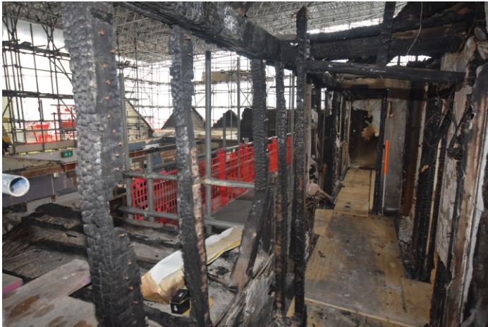
Plate 52: First Floor Corridor AA, looking to right
