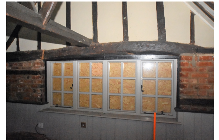
Plate 41: Room I window to front
