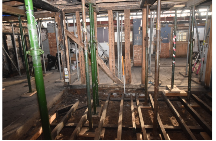
Plate 22: Room E, wooden stud 'screen' to rear
