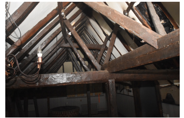
Plate 33: Room I truss
