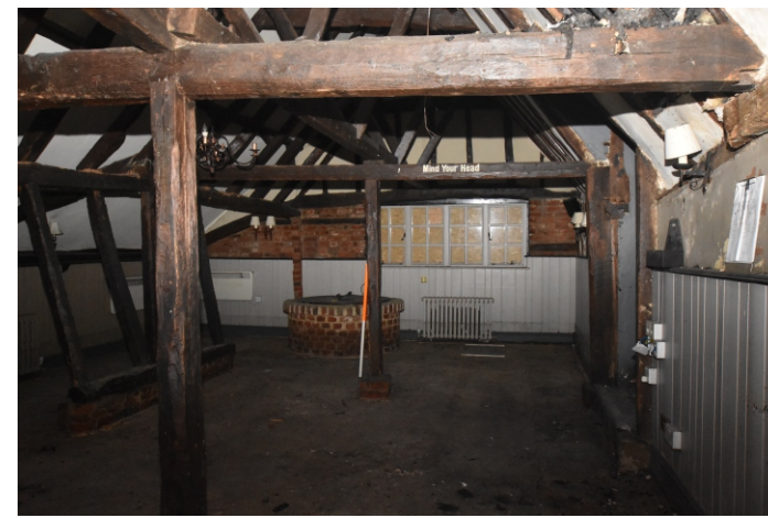
Plate 32: Room I looking to front
