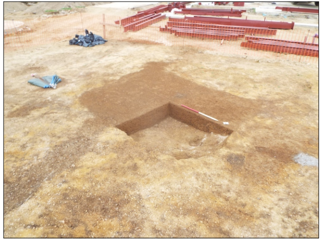
Photograph 4: SFB 1 Looking East, Showing Sections 046 and 047
