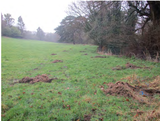
PHOTOGRAPH 1: SOUTHERN END OF TREE PLANTING AREA LOOKING NORTH, AFTER EXCAVATION OF TREE PLANTING PITS
