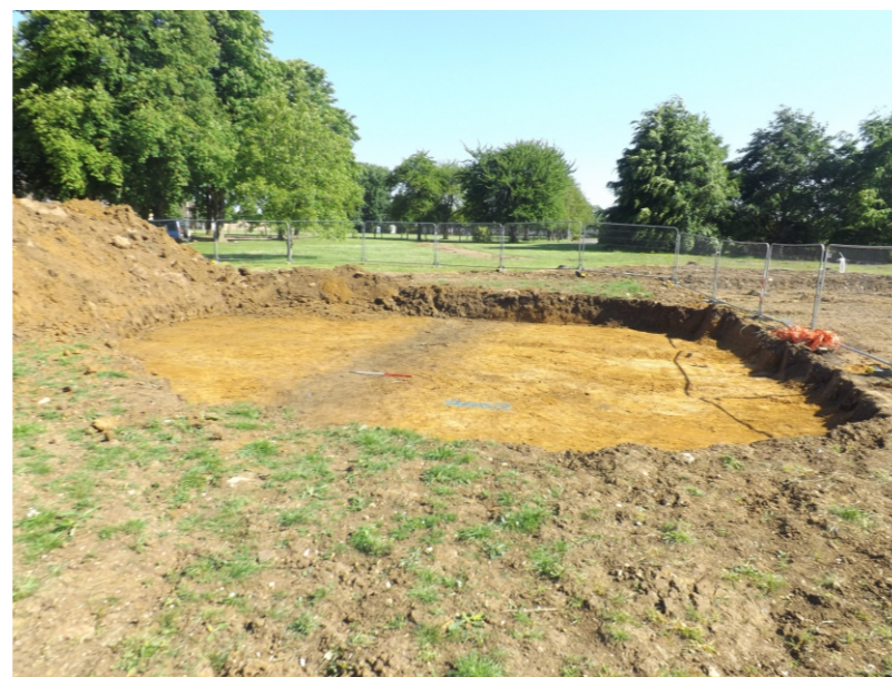
PHOTOGRAPH 5: AREA 2 LOOKING NORTH
