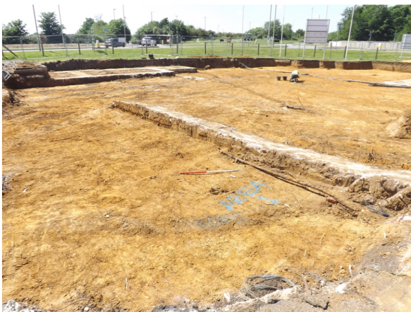
PHOTOGRAPH 4: AREA 1 LOOKING SOUTHWEST
