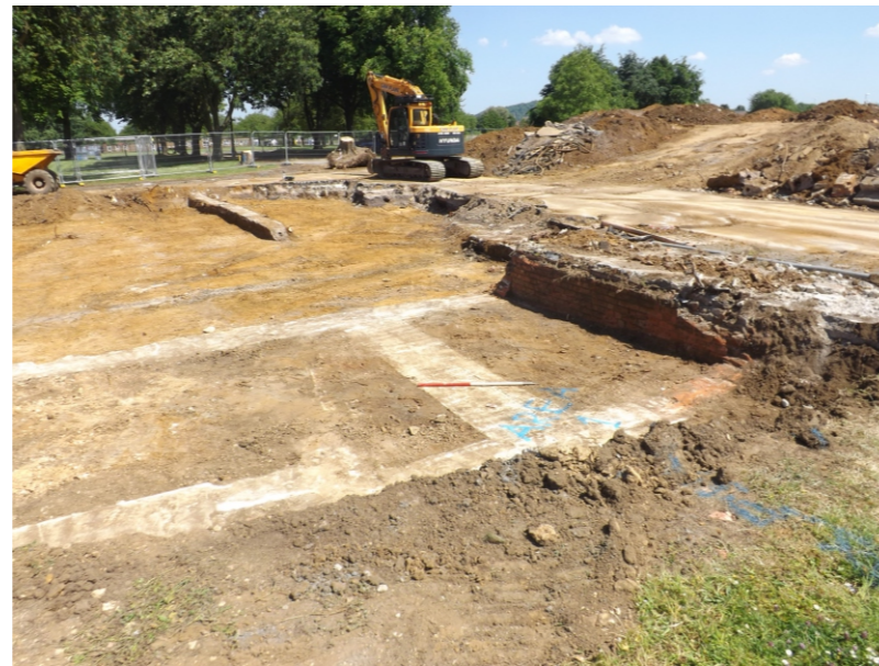
PHOTOGRAPH 2: AREA 1 LOOKING NORTHEAST
