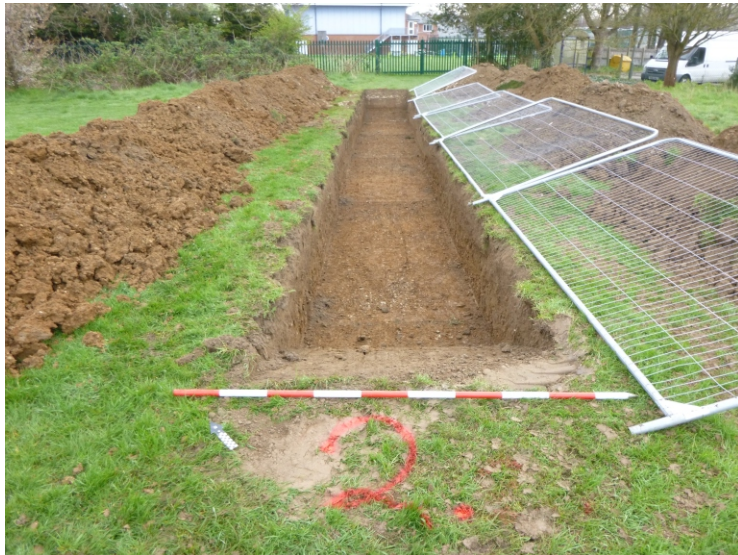
Trench 2. Looking Northeast
