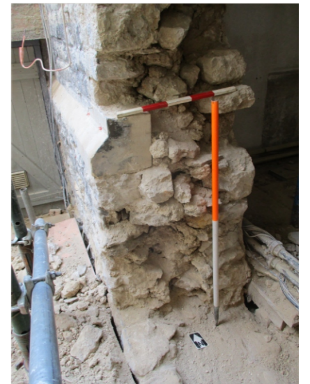
PHOTOGRAPH 13: DETAIL OF SOUTH FACING WALL SECTION
