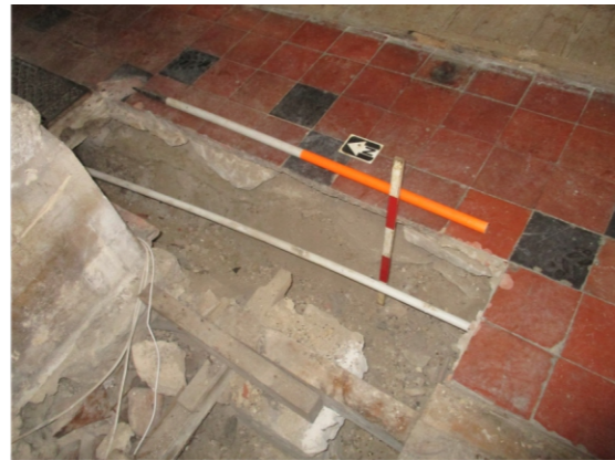
PHOTOGRAPH 6: SERVICE TRENCH C, LOOKING NORTHEAST
