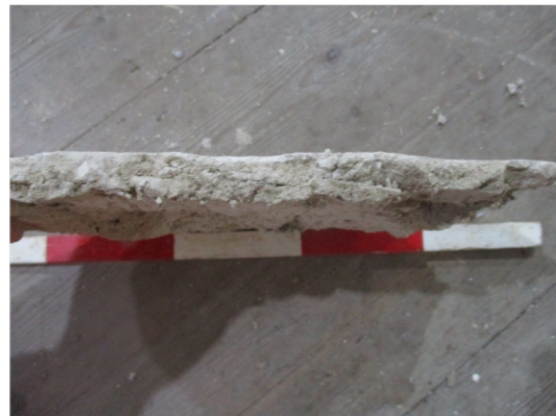
PHOTOGRAPH 10: FRAGMENT OF INTERIOR WALL RENDER
