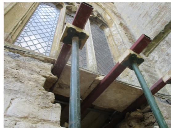
PHOTOGRAPH 16: TOP OF WALL EXCAVATION, SHOWING BASE OF WINDOWSILL STONE SLABS
