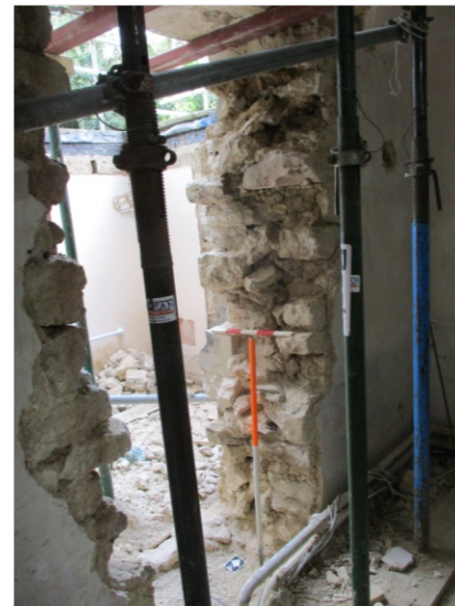
PHOTOGRAPH 12: SOUTH FACING WALL SECTION
