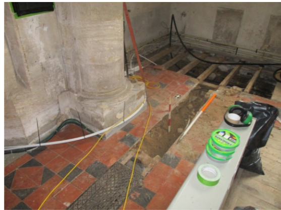
PHOTOGRAPH 5: SERVICE TRENCH B, LOOKING NORTHWEST
