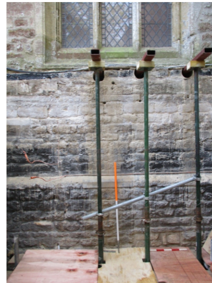
PHOTOGRAPH 8: EXTERIOR WALL ELEVATION, PRIOR TO REMOVAL
