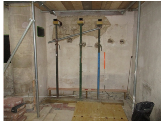
PHOTOGRAPH 7: INTERIOR WALL ELEVATION, PRIOR TO REMOVAL
