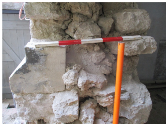
PHOTOGRAPH 14: DETAIL OF CHAMFERED STONE IN SOUTH FACING WALL SECTION
