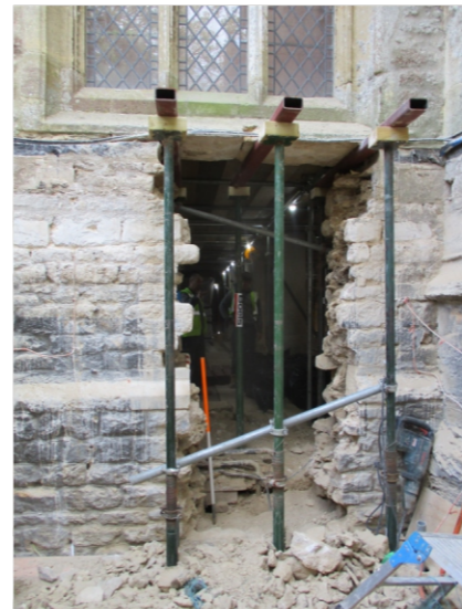
PHOTOGRAPH 11: EXTERIOR VIEW AFTER WALL REMOVAL
