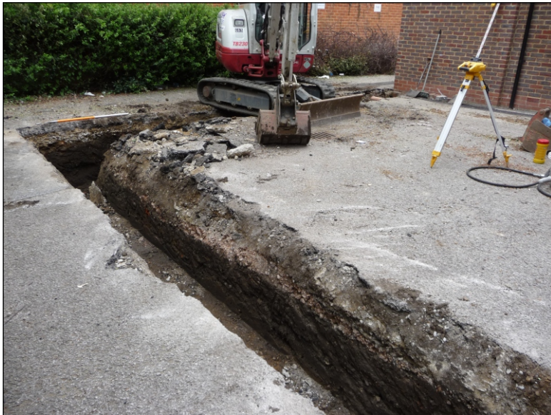
Plate 3: Site photograph, looking south
