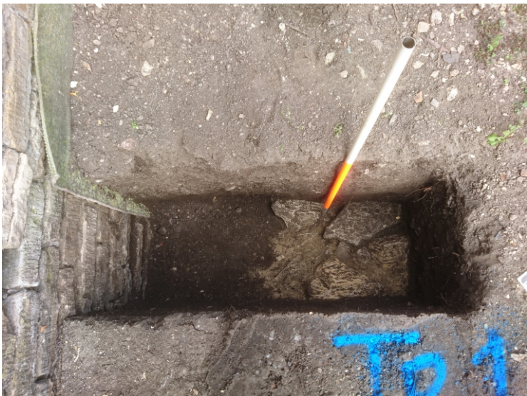
Overhead Shot of Test Pit 1
