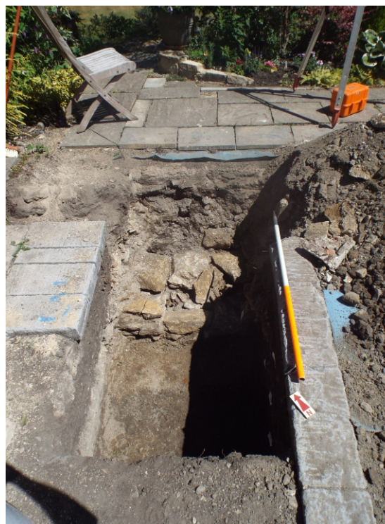
Test Pit 5 Looking Northeast
