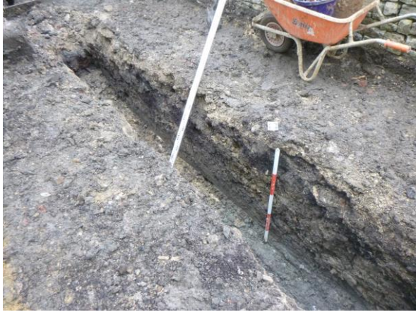
Photograph 2 – representative section of foundation trench
