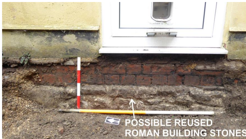
Photograph 1: Partly exposed house footings showing possible reused Roman building stones
