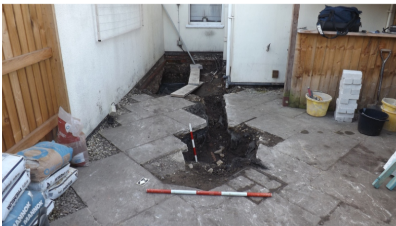
PHOTOGRAPH 1: GROUNDWORKS EXCAVATIONS LOOKING SOUTHEAST
