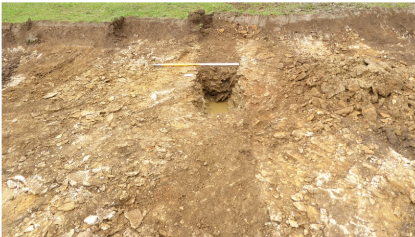
PHOTOGRAPH 2: DRAIN 1 (SECTION 1), LOOKING WEST. EXCAVATION ABANDONED DUE TO FLOODING
