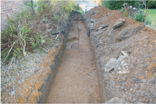
TRENCH 1 LOOKING WEST
