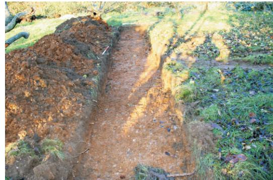
TRENCH 4 LOOKING NORTHEAST
