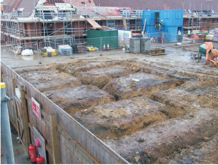
WEST FACING SHOT OF PLOT 56, EXCAVATED
