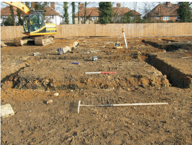
EAST NORTHEAST FACING SHOT PLOT 53, EXCAVATED
