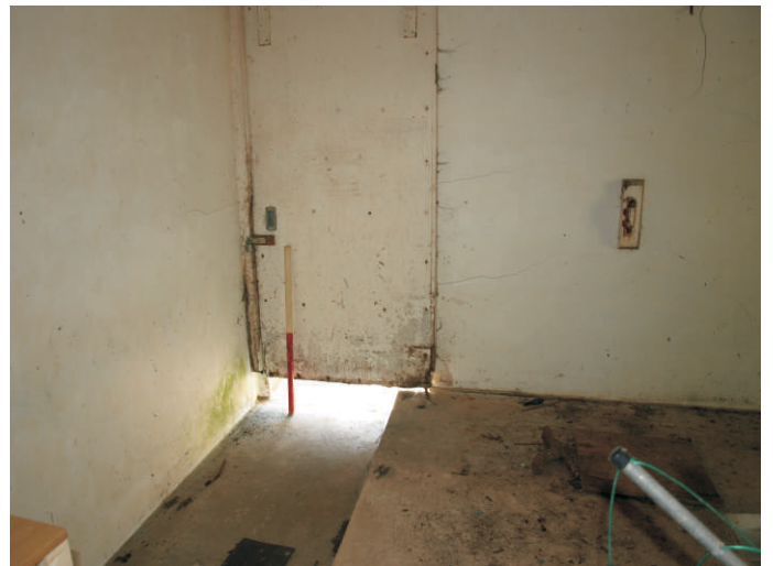
MAIN ROOM, FEEDING TROUGH DETAIL
