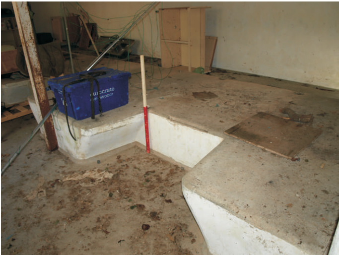
MAIN ROOM, MILKING STALL DETAIL
