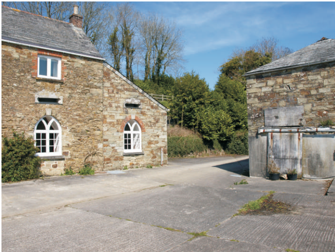
THE FARMER'S HOUSE ON THE LEFT THE SOUTHWEST ELEVATION OF THE BARN ON THE RIGHT
