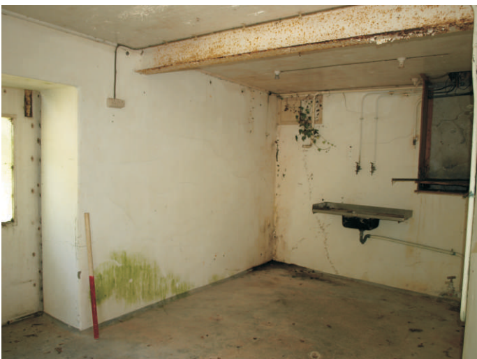
NORTHEAST ROOM, EAST FACING
