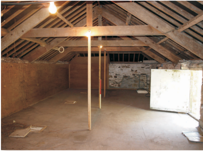
INTERNAL, FIRST FLOOR, SOUTHWEST FACING
