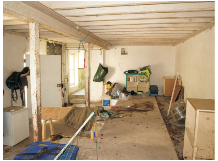
MAIN ROOM, NORTHEAST FACING
