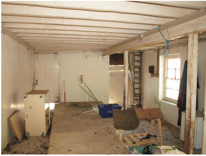
MAIN ROOM, SOUTHWEST FACING
