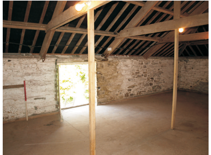
INTERNAL, FIRST FLOOR, NORTHWEST FACING
