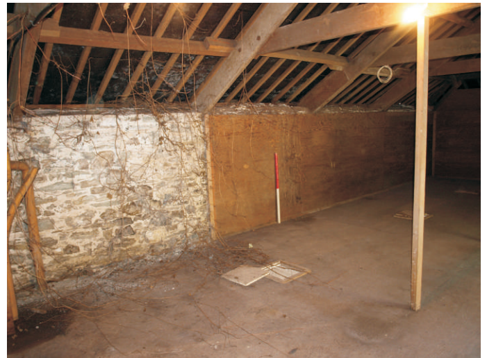
INTERNAL, FIRST FLOOR, SOUTH FACING
