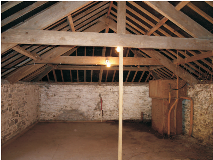
INTERNAL, FIRST FLOOR, NORTHEAST FACING
