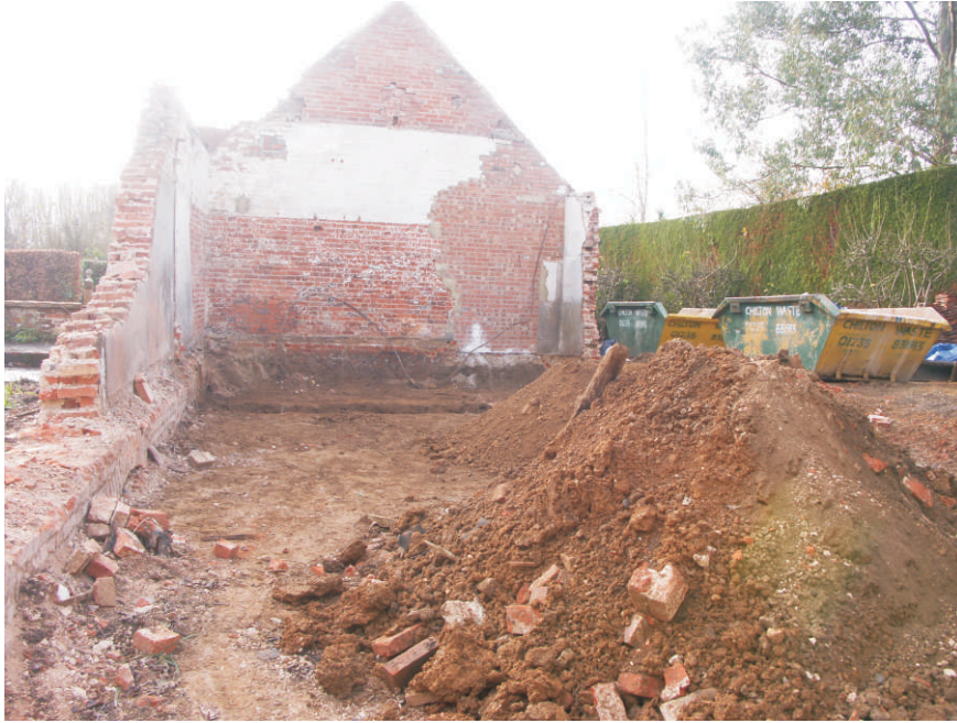
SOUTH FACING SHOT OF EXCAVATED AREA
