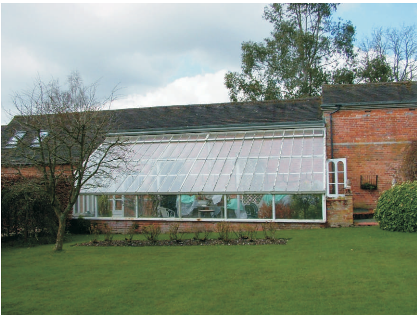
WEST FACING SHOT OF THE REAR (EAST FACING ELEVATION) OF THE NORTHERN END OF MANOR FARM HOUSE BEFORE COMMENCEMENT OF WORKS. THE SITE IS SITUATED ON THE RIGHT OF THE PHOTOGRAPH. THE GLASS BUILT BUILDING (CONSERVATORY) WAS ALSO SUBSEQUENTLY DEMOLISHED.
