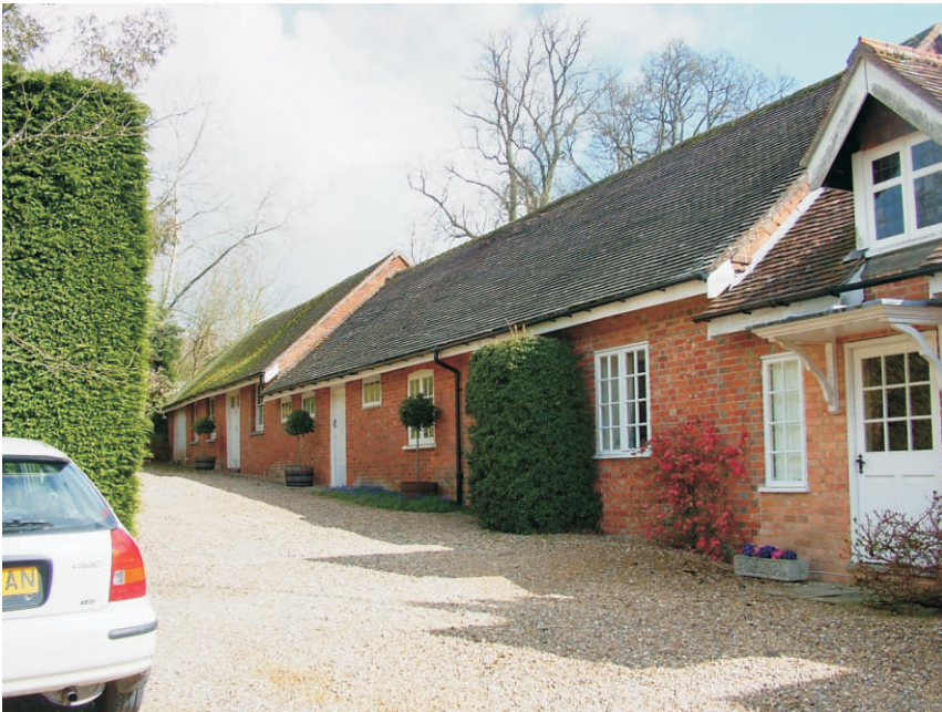
NORTHEAST FACING SHOT OF FRONT (WEST FACING ELEVATION) OF MANOR FARM HOUSE BEFORE COMMENCEMENT OF WORKS. THE SITE IS SITUATED AT THE 'BACK' OF THE PHOTOGRAPH
