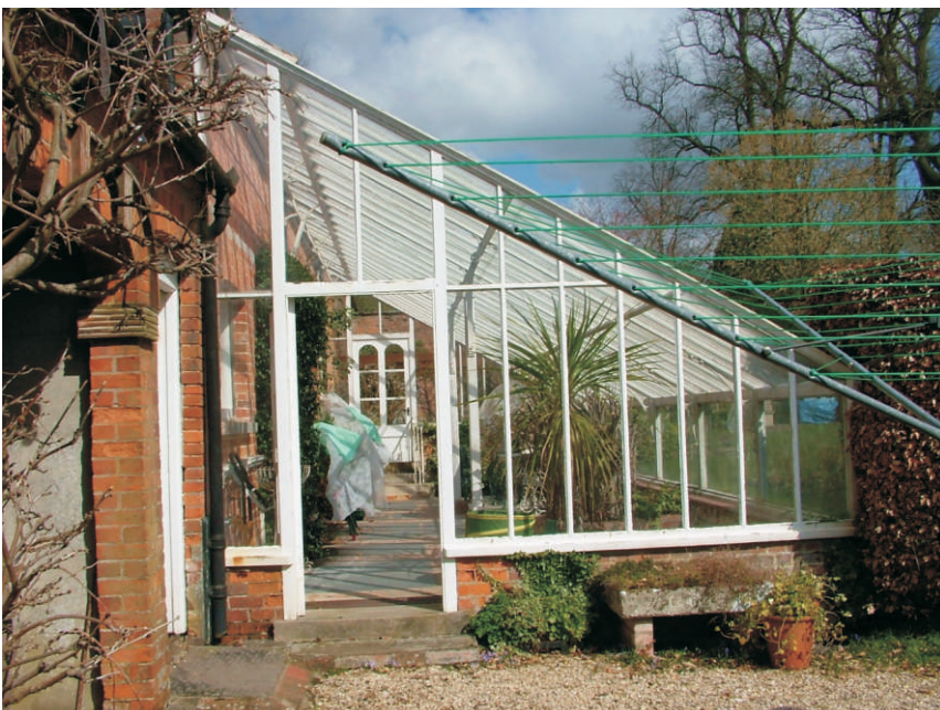
NORTH FACING SHOT OF THE CONSERVATORY BEFORE COMMENCEMENT OF WORKS.
