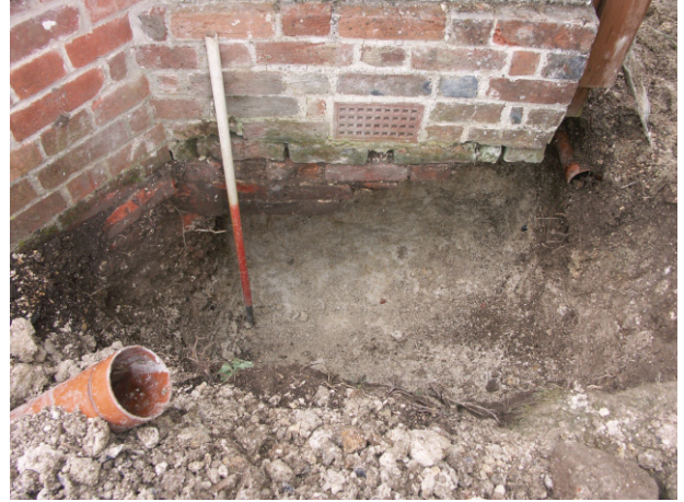
Northeast facing shot of Bay 1, fully excavated.
