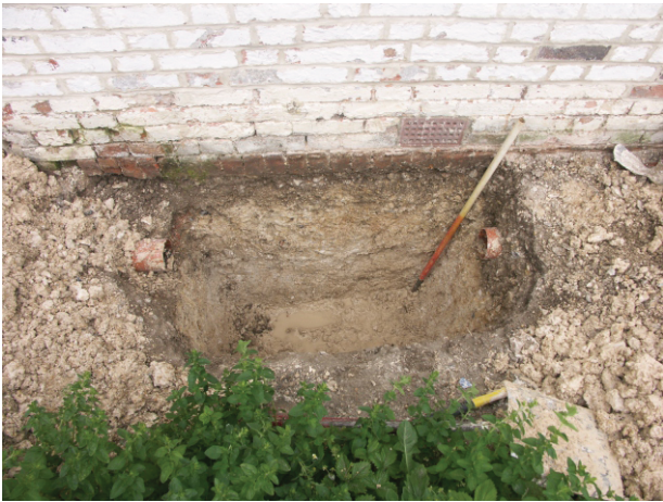
Northwest facing shot of Bay 5, partially excavated.
