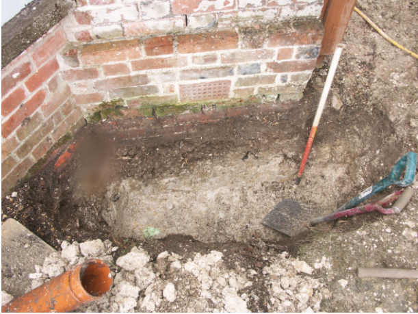
Northeast facing shot of Bay 1, partially excavated.
