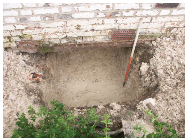
Northwest facing shot of Bay 5, fully excavated.
