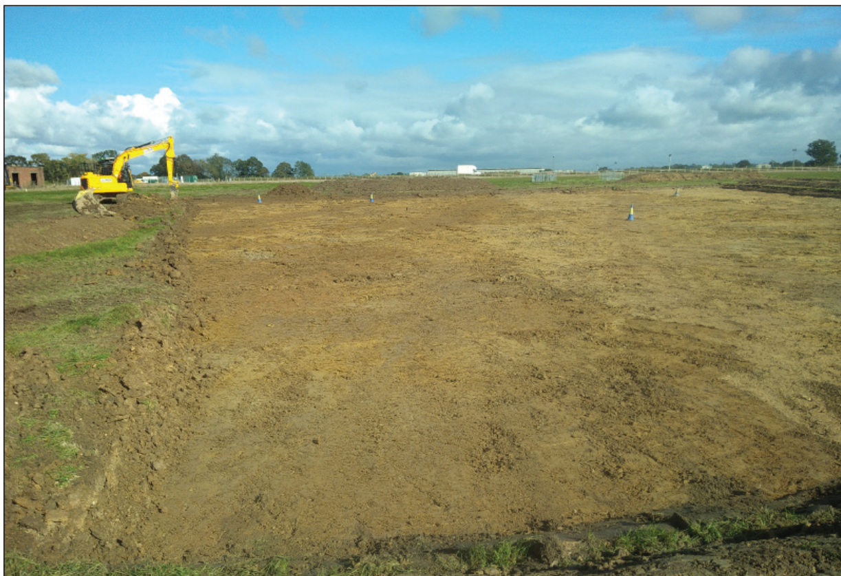
Plate 3 - Working shot, Trench 32
