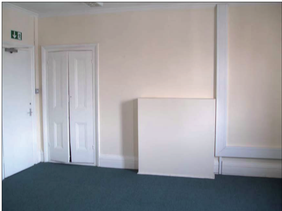
Plate 10: Original built in cupboard and possible concealed fire place on second floor
