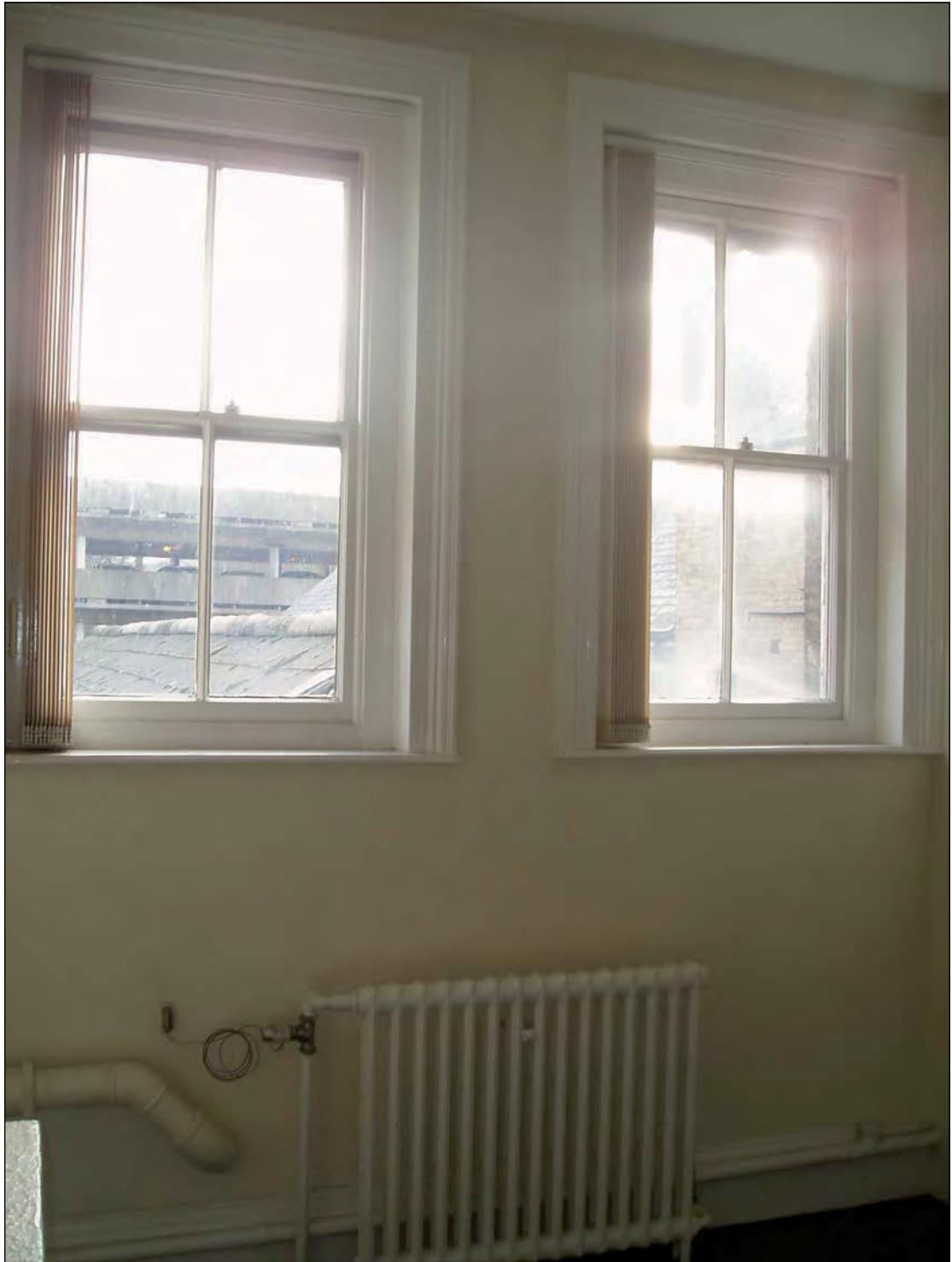
Plate 6: Original windows on first floor
