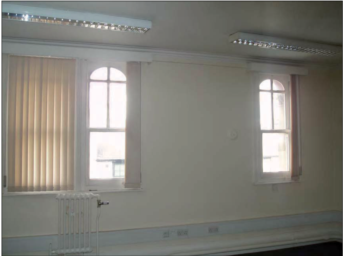
Plate 7: Original windows on second floor
