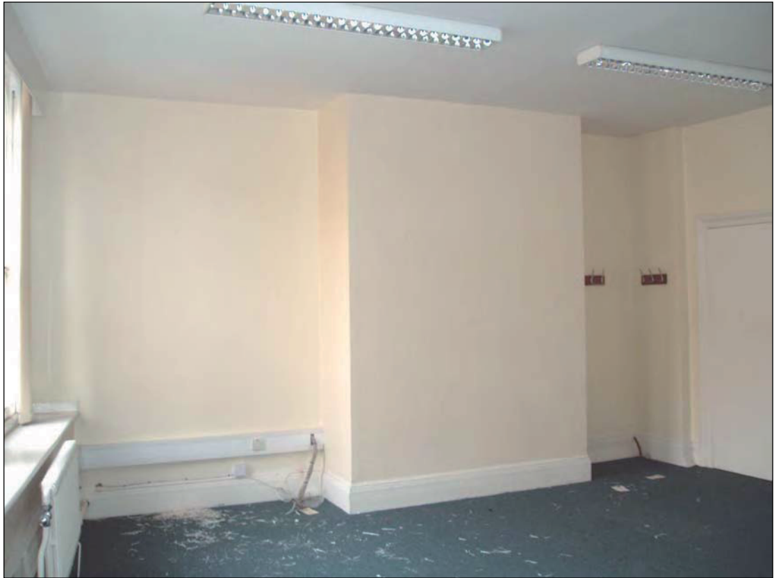
Plate 9: Possible concealed fireplace on first floor
