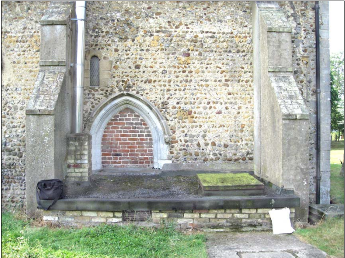
Plate 15: Sunken boiler room
