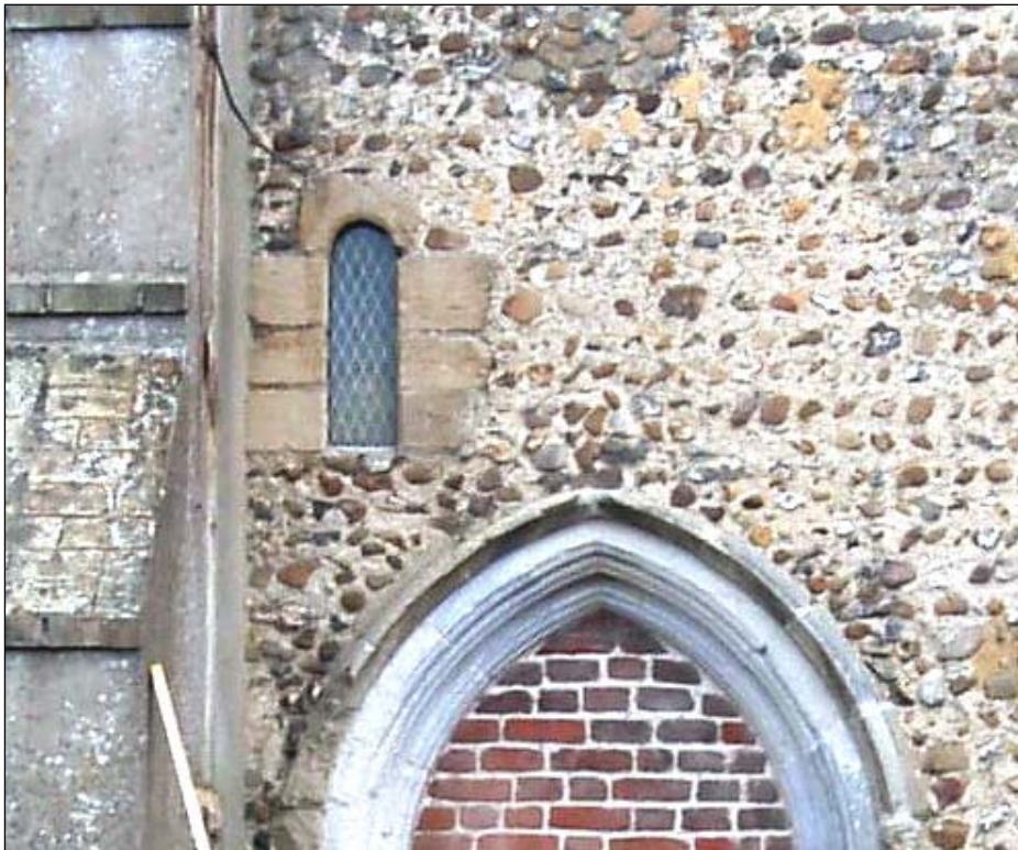
Plate 16: Norman window in north wall
