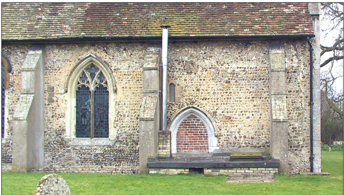
Plate 14: North-facing wall of church, prior to work
