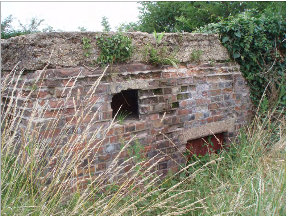
Plate 2: Access door on south-west elevation
