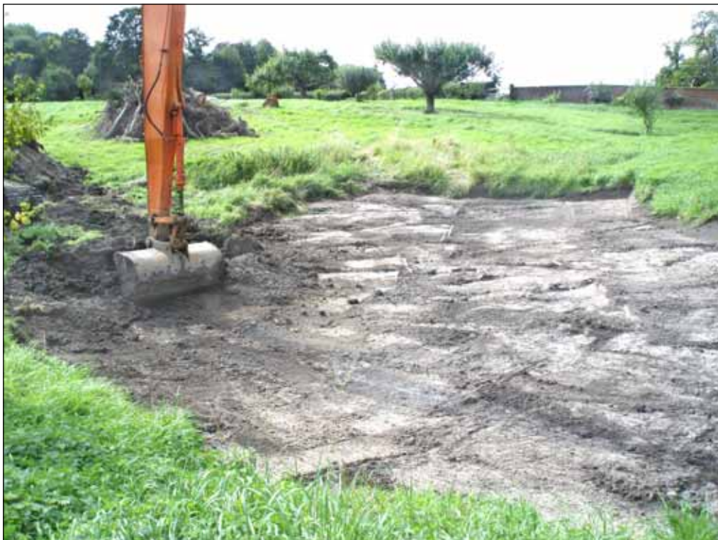
Plate 4: Excavation of Horse Pond in progress, facing south-west.
