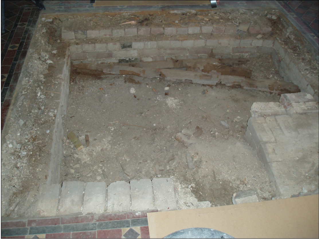
Plate 2: Brick walls for supporting former wooden pews and around base of medieval column
