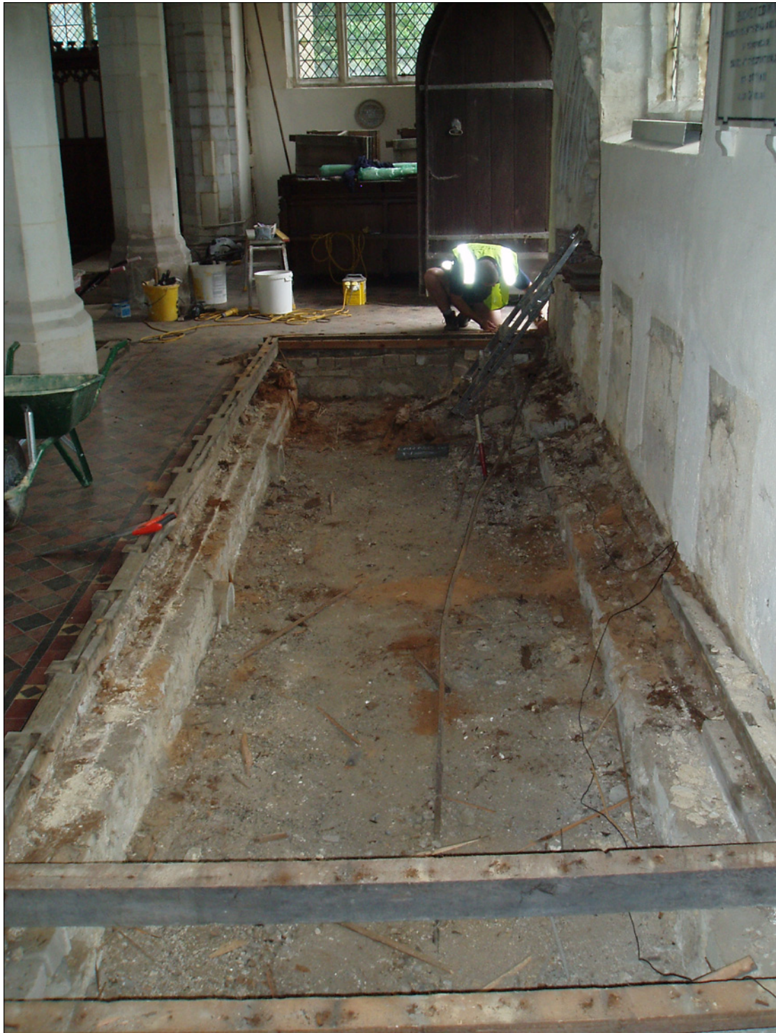
Plate 1: Stones walls remaining after removal of pews in north transept
