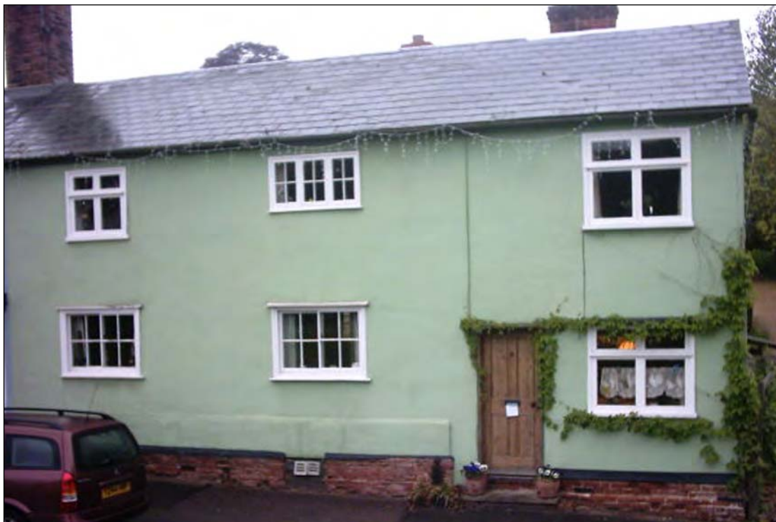
late 2 : Front of 2 High Street
