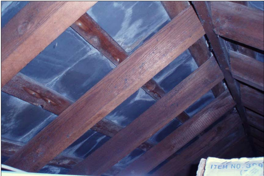
late : epla ed roof
