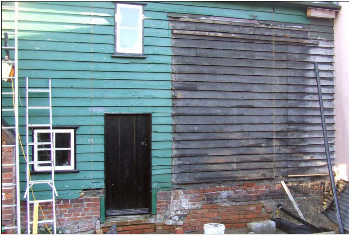
late 3: weather boarding following removal of lean to
