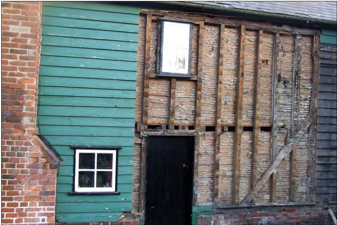
late 4: timber frame exposed following removal of weather boarding
