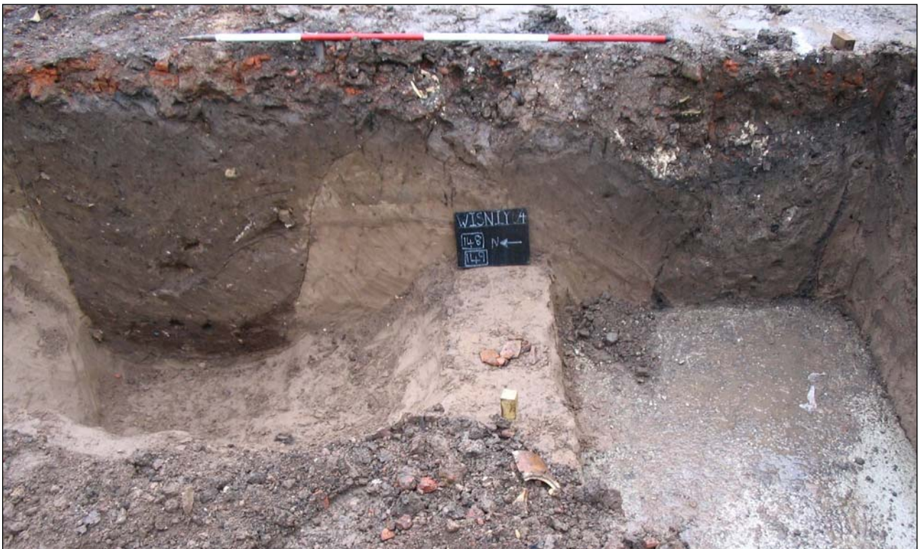
Plate 4: Section 14, pit 148 (excavated) and pit 149 (with concrete foundation poured)
