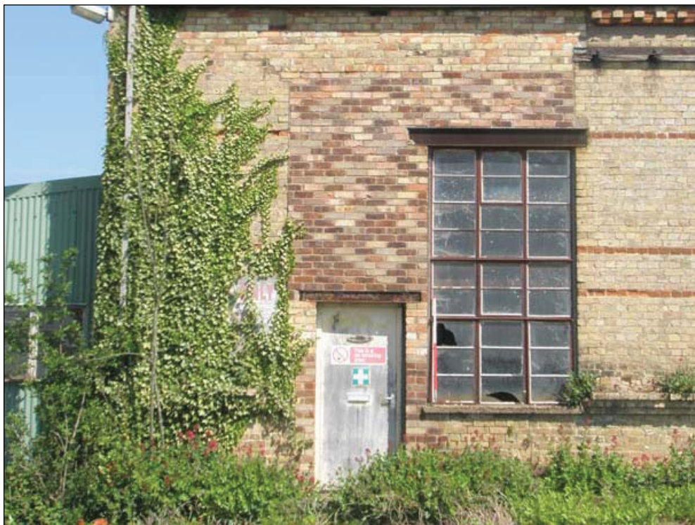
Plate 19: Blocked opening on south facing elevation of Building F
