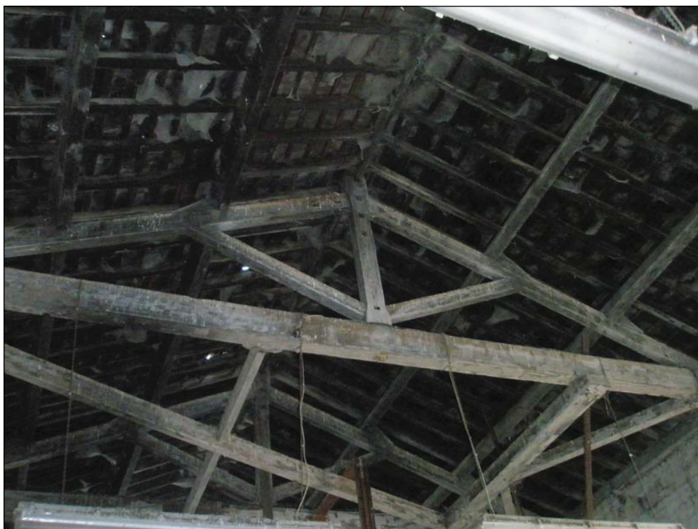
Plate 23: Detail of king post and tusk tenon roof structure in Building F
