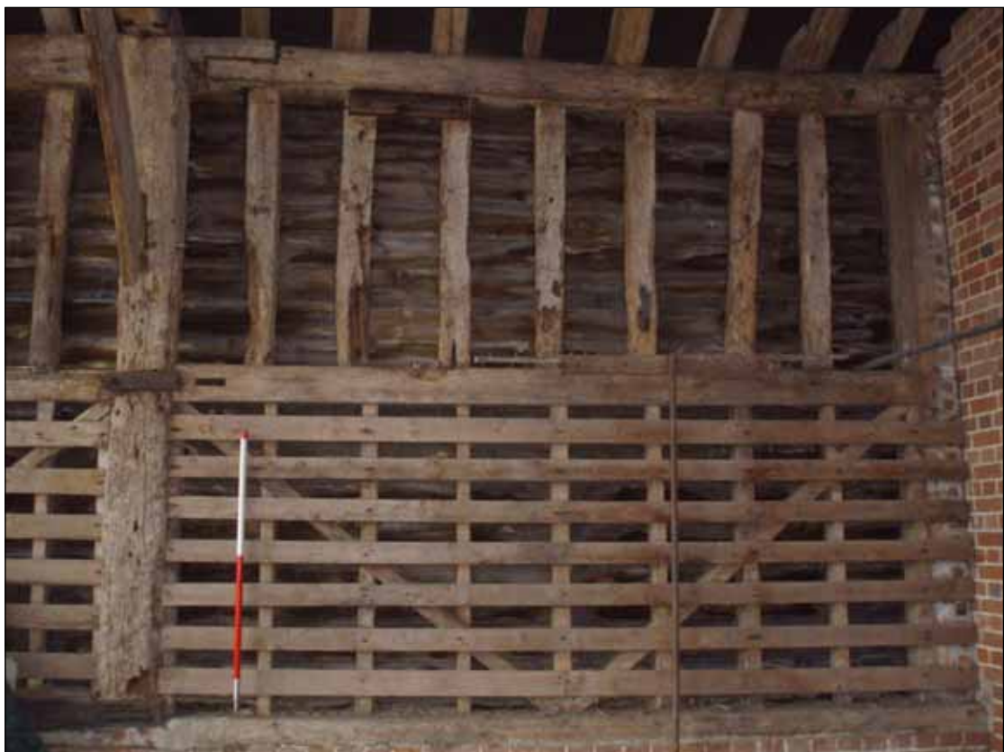
Plate 20: Building 7 internal detail
