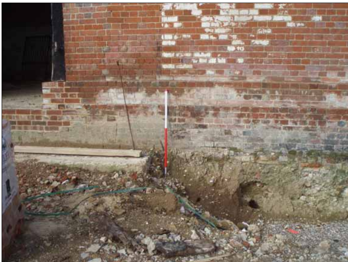
Plate 25: Footings for threshing barn exposed during groundworks
