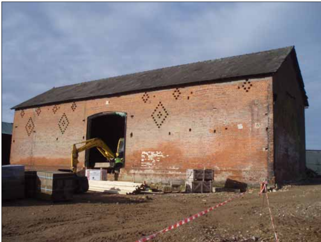
Plate 1: East facing elevation of threshing barn
