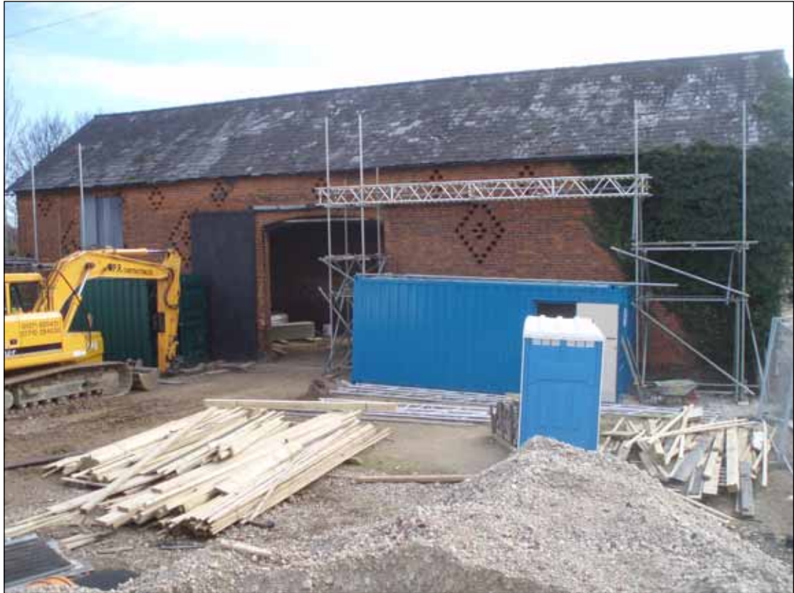
Plate 7: West facing elevation of threshing barn
