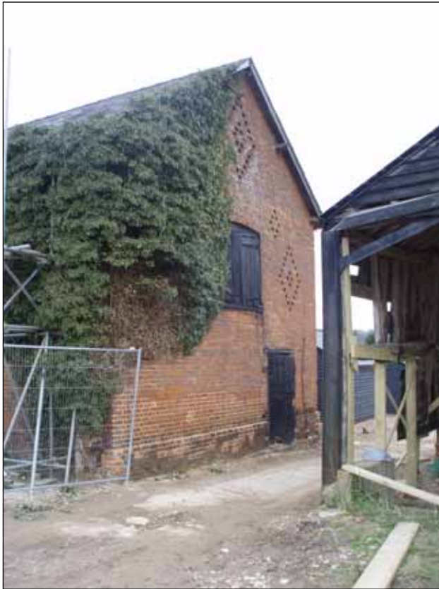
Plate 5: South facing elevation of threshing barn
