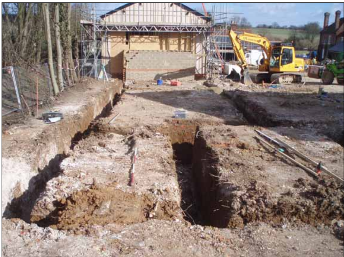
Plate 24: Footings for extension to building 2
