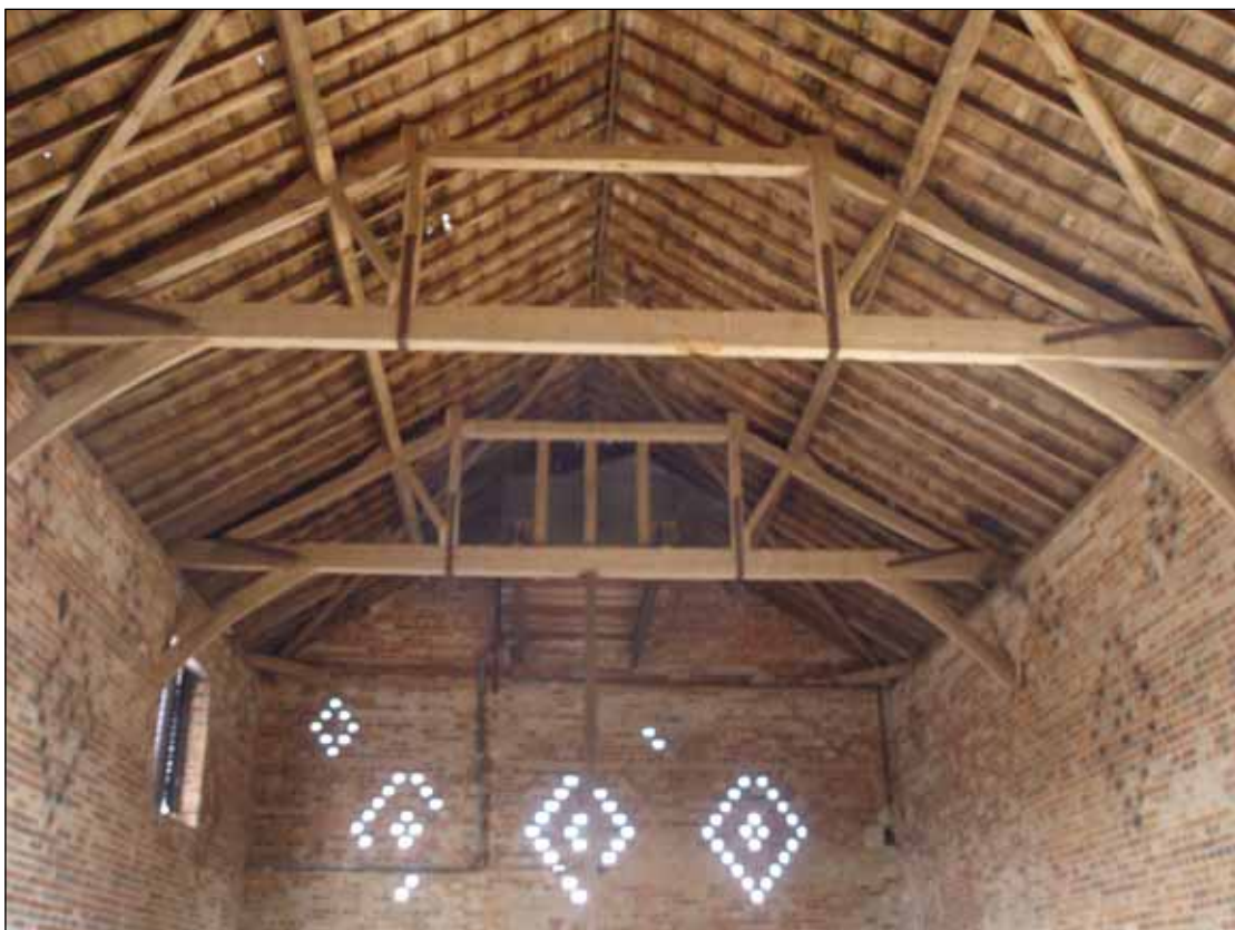
Plate 10: Roof construction of threshing barn
