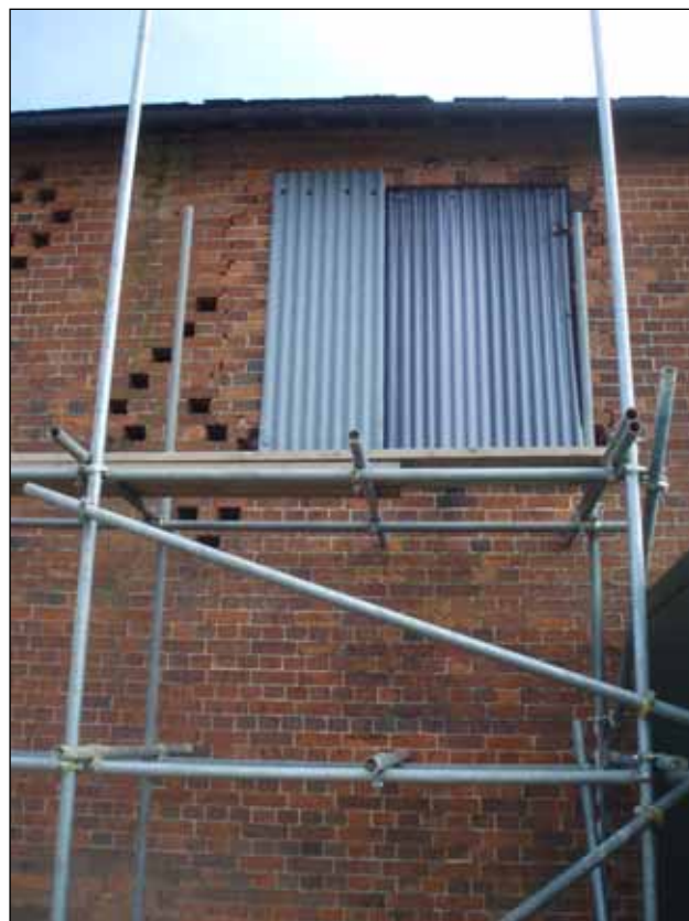
Plate 8: Inserted opening in west facing elevation
