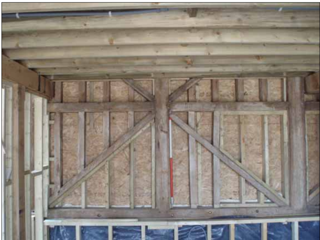
Plate 12: Detail of inside building 2
