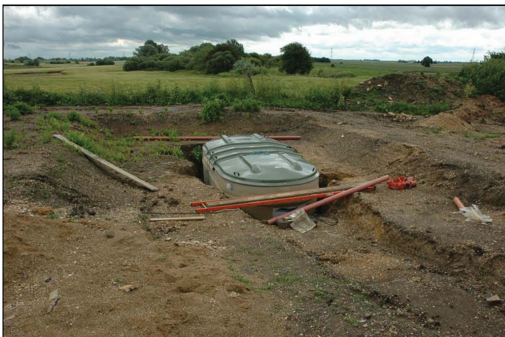
Plate 1: Watching brief trench following insertion of tank (Copyright Ben Robinson, by permission)
