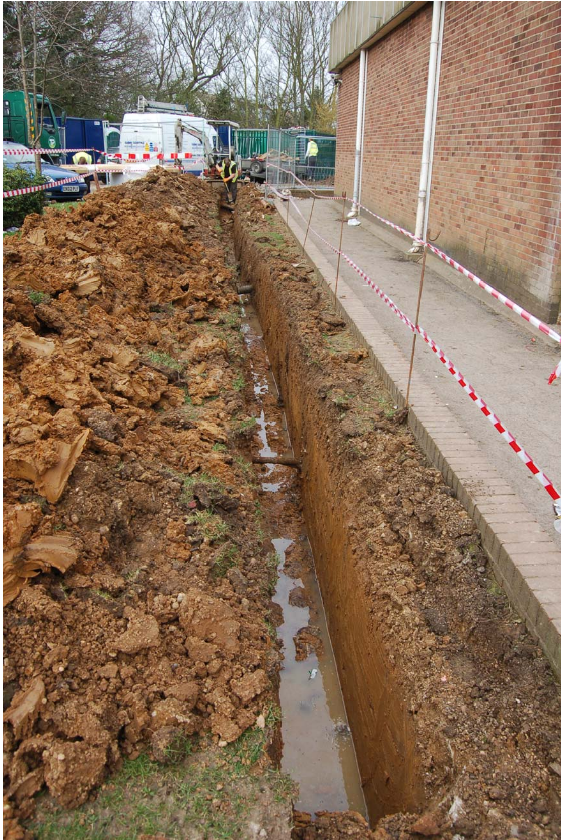
Plate 3: View of service trench looking south
