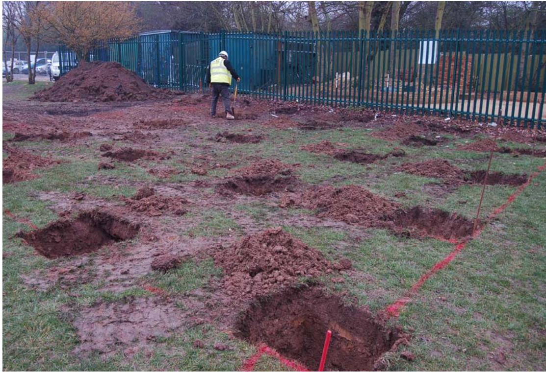
Plate 1: General view of post-pads under excavation
