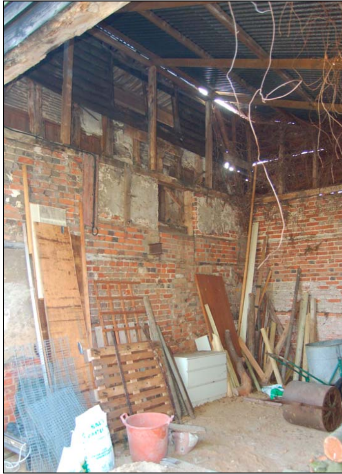
Plate 5 South-west wall of granary and former kiln interior
