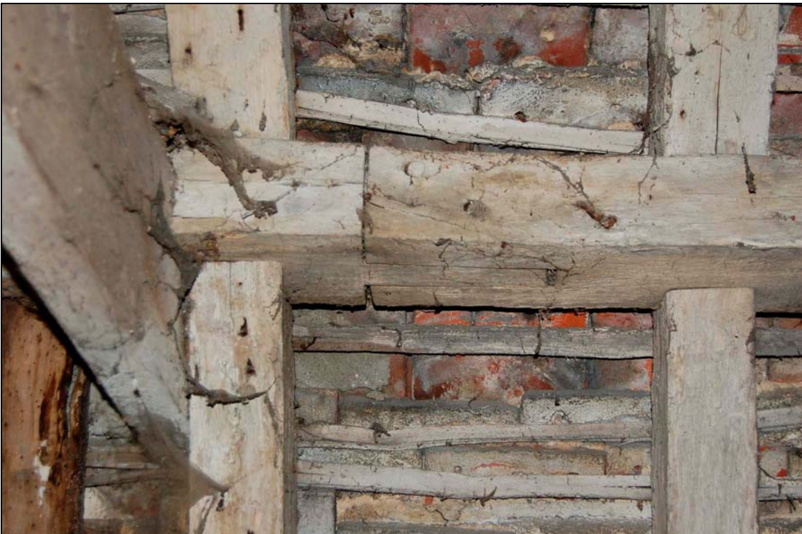
Plate 14 Plain scarf joint in wall plate
