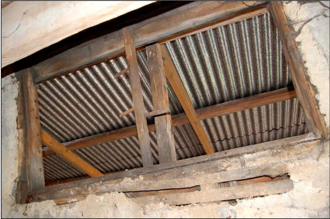
Plate 15 Former vent at south-west end of granary
