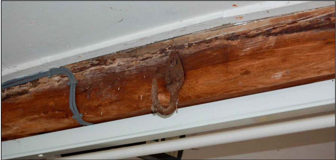
Plate 9 Iron hook on bridging joist in garage
