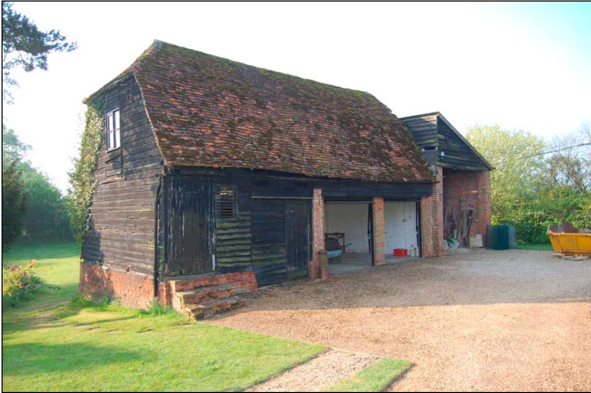
Plate 1 Granary viewed to south
