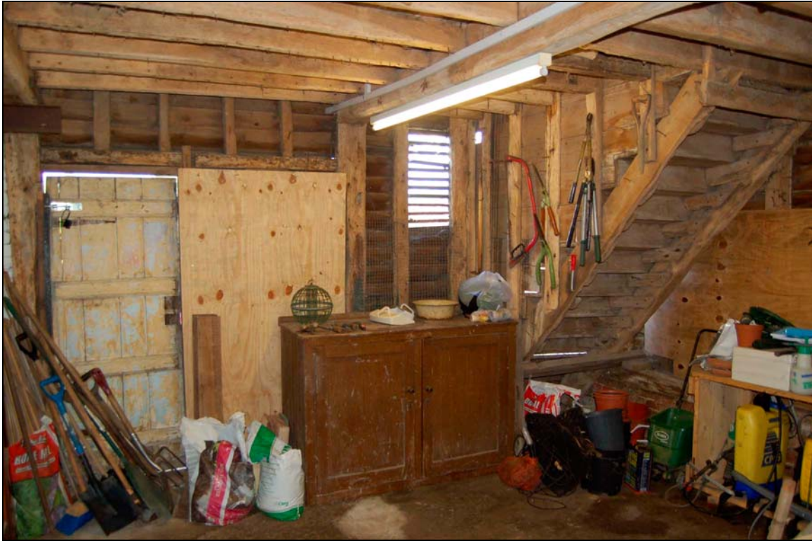
Plate 7 Interior of garden store viewed to north-west
