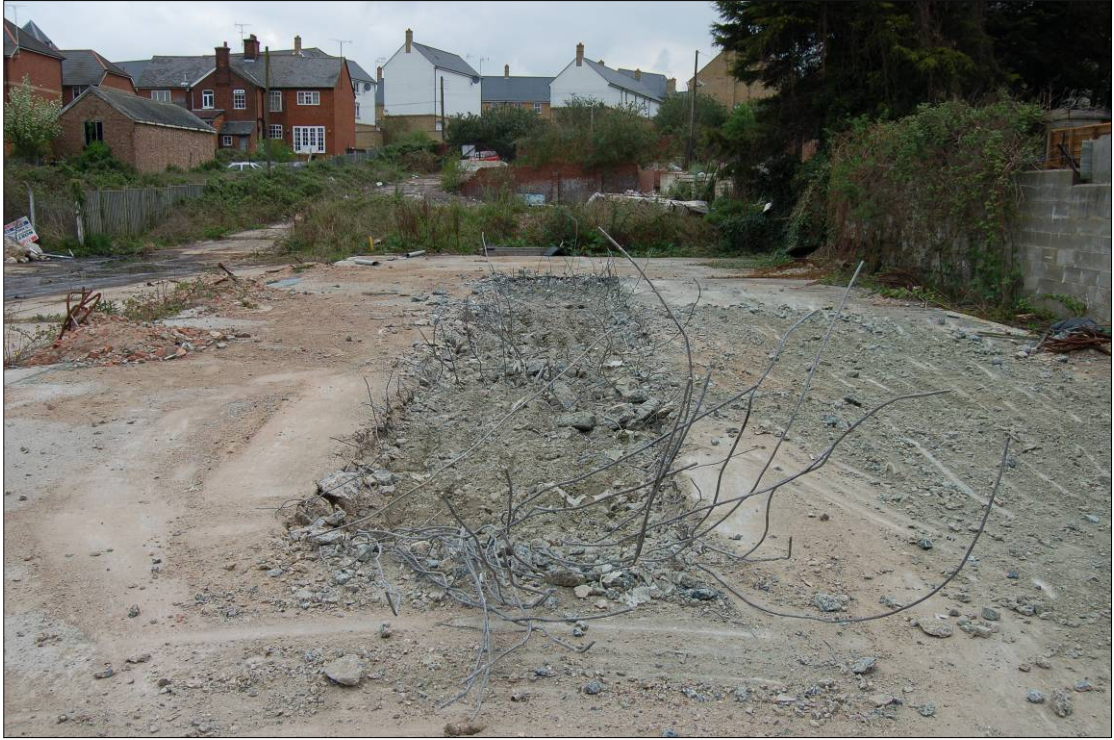
Plate 13: Trench 10 – view of reinforced concrete floor slab looking north
