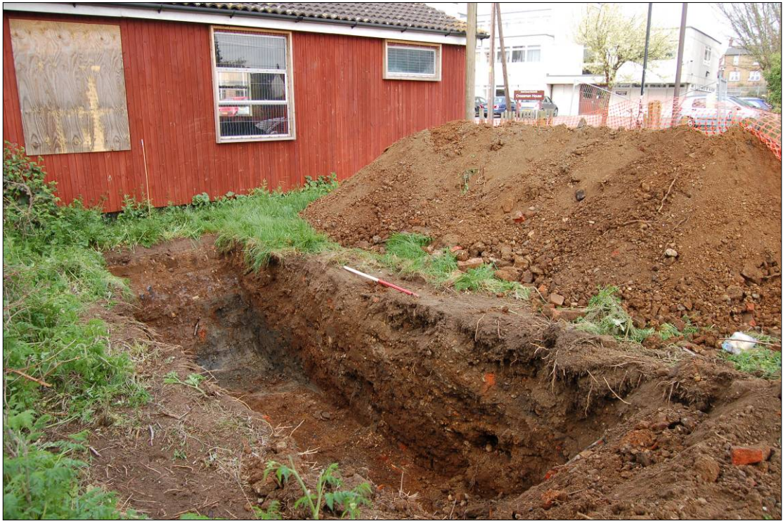
Plate 1: Trench 1 looking north west (1m scale)
