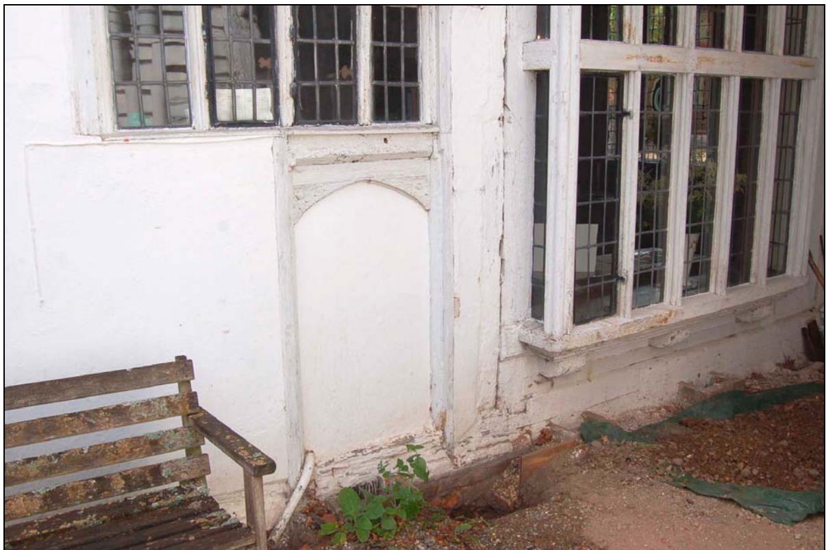
Plate 4 Location of test-pit 3 in passage
