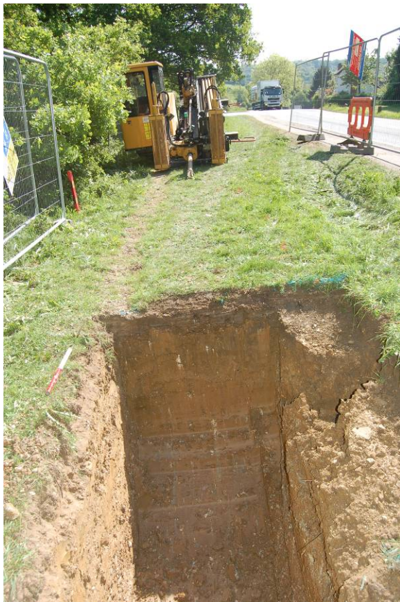
Plate 1. Pit 1 (looking east)
