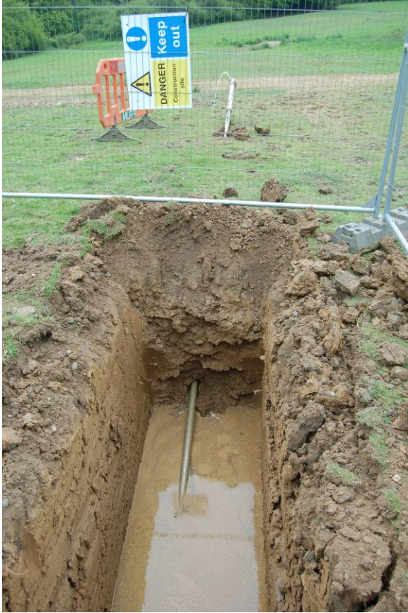
Plate 4. Pit 8 after drilling (looking east)
