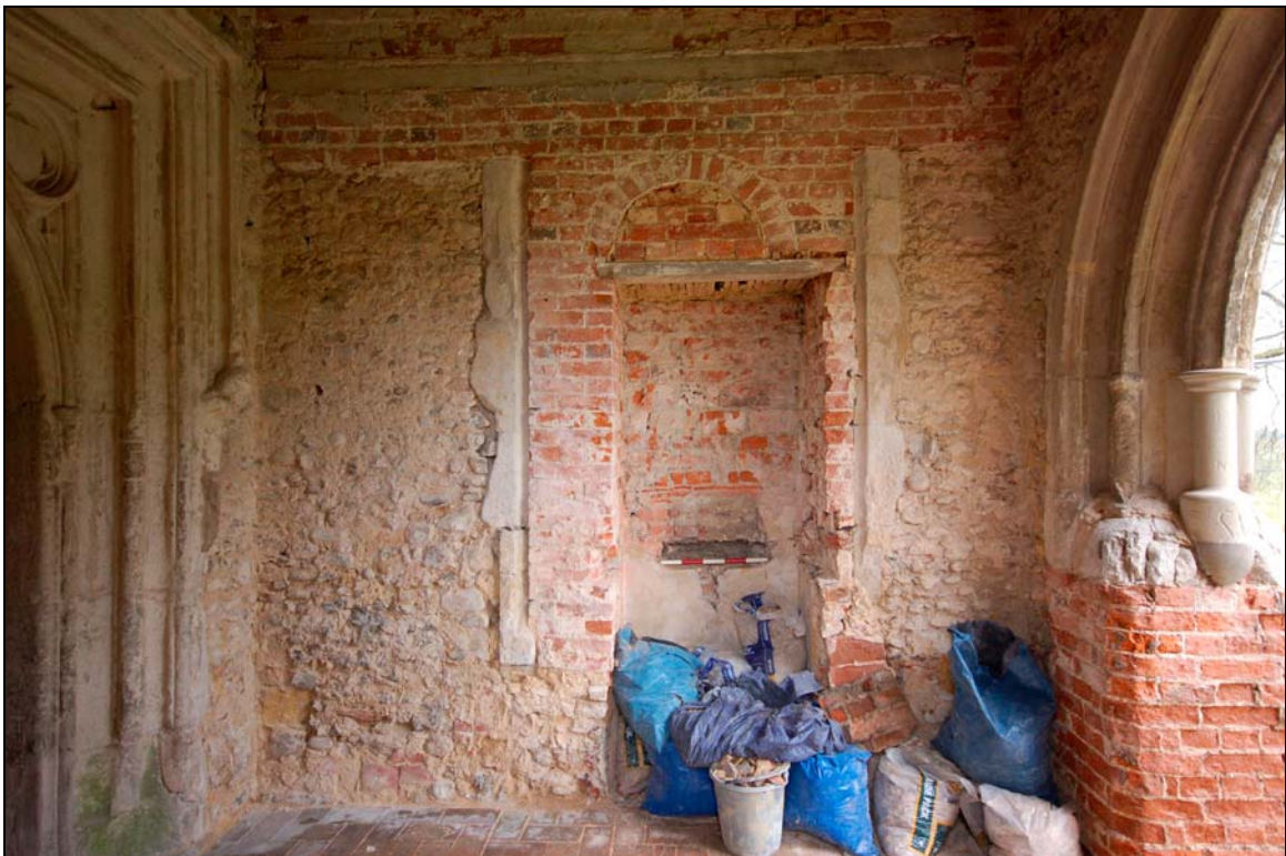
Plate 6 Exposed 15th and 18th-century windows on eastern wall
