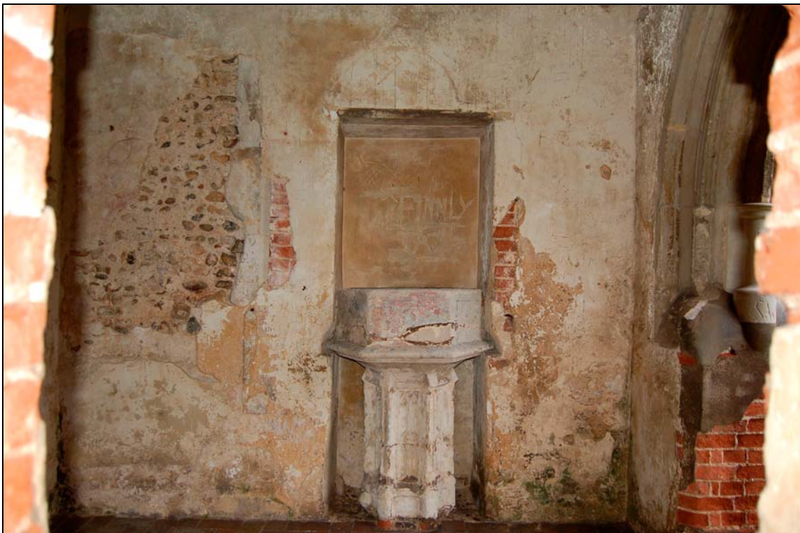
Plate 4 East wall of porch before start of works
