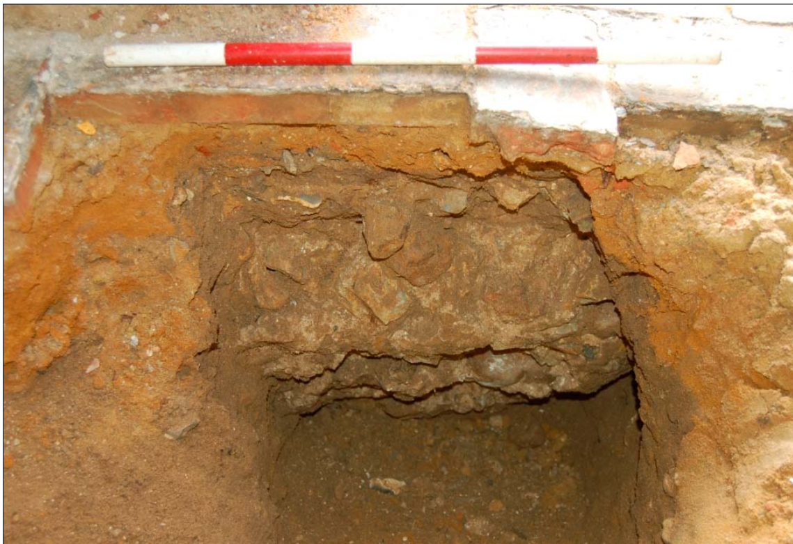
Plate 8 Internal foundation exposed in exploratory pit looking south (0.5m scale)
