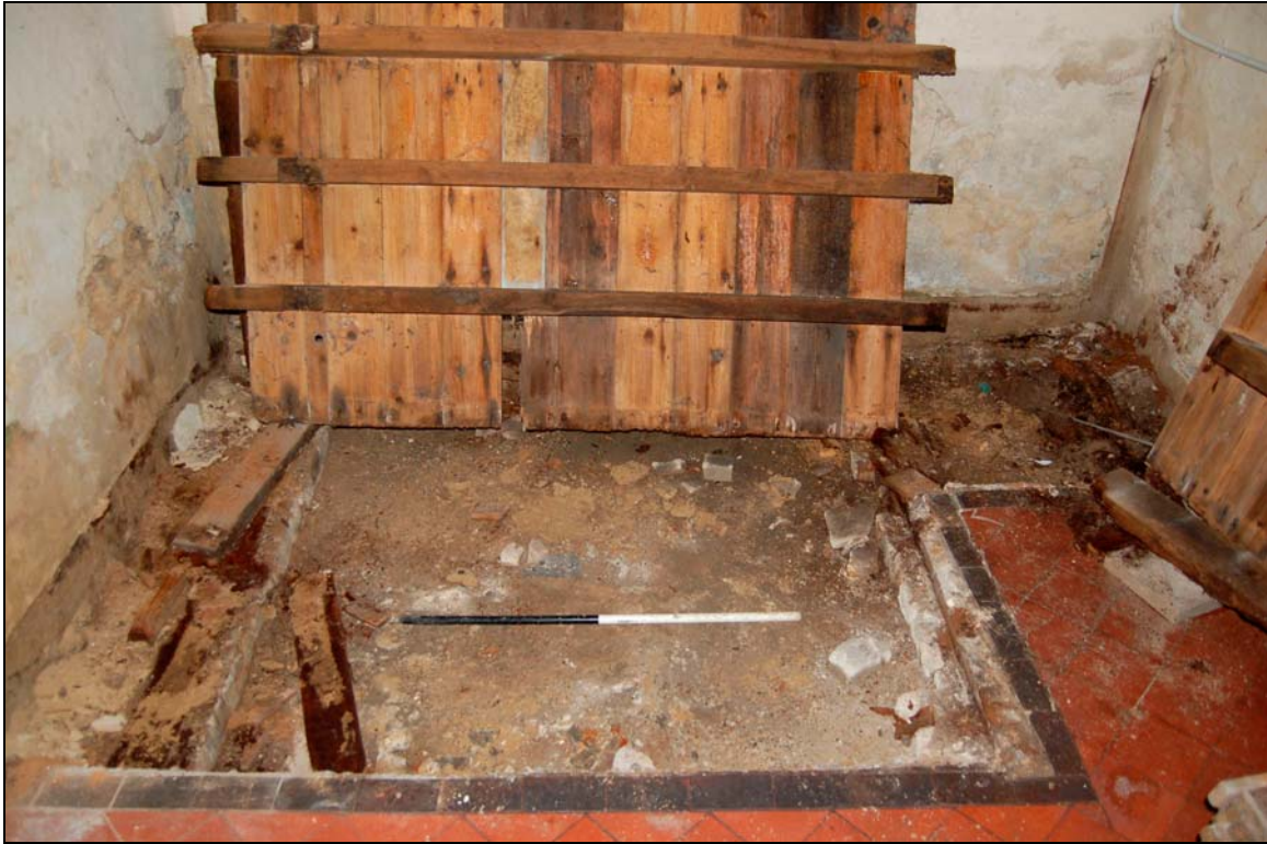
Plate 7 Area of removed flooring
