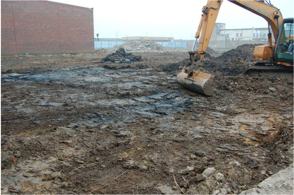
Plate 1 and 2: Levelling following the removal of hardstanding, Block C
