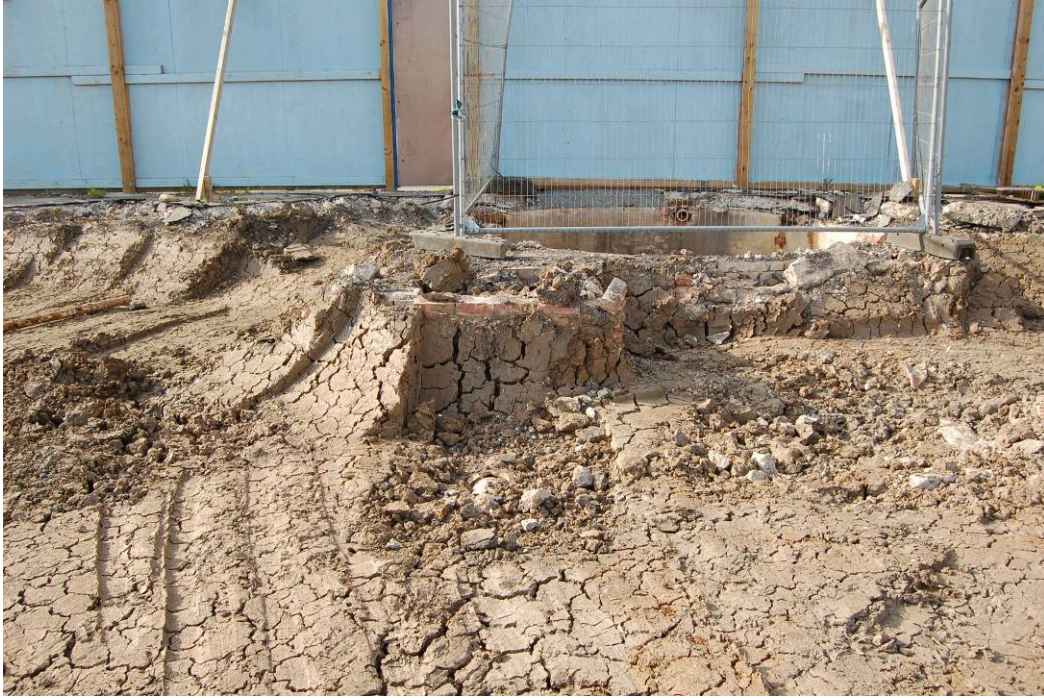
Plate 3: Concrete lined access to drains, located on the frontage between Block D and E
