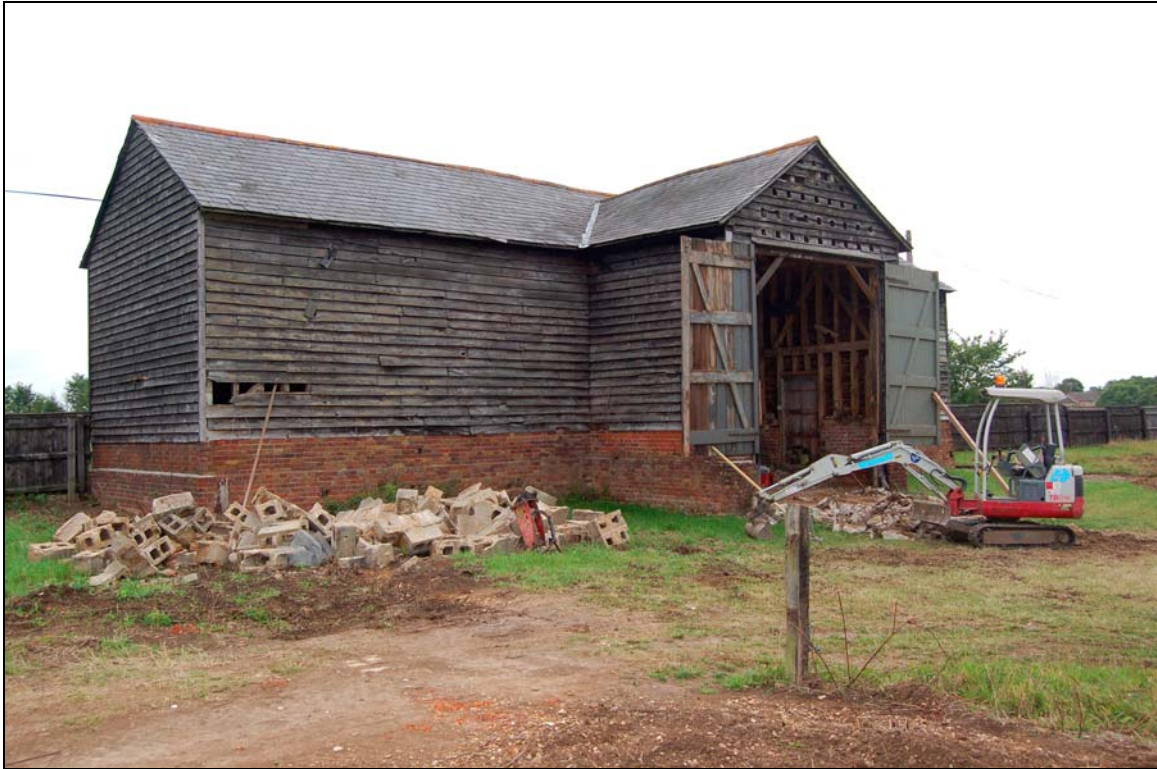
Plate 1 Barn 1 viewed to north-east from yard
