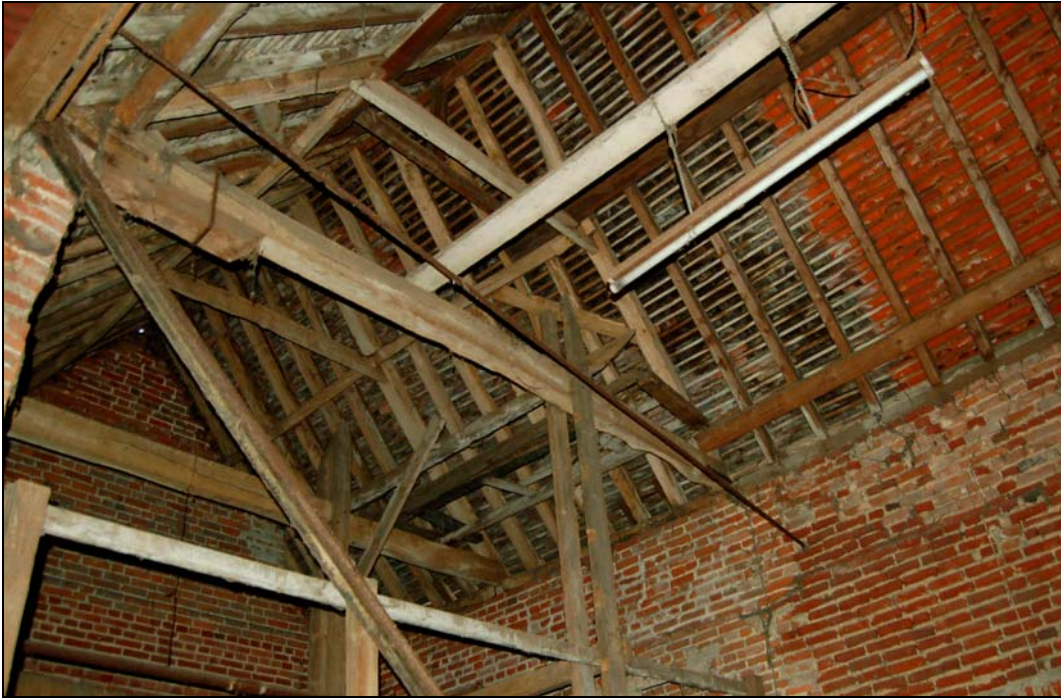
Plate 9 Original roof frame in northern bays
