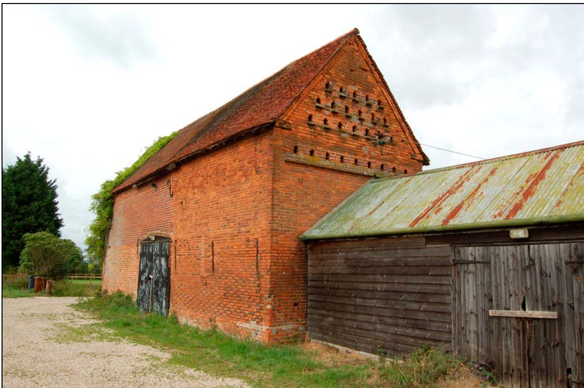
Plate 6 Rebuilt eastern wall and northern dovecote
