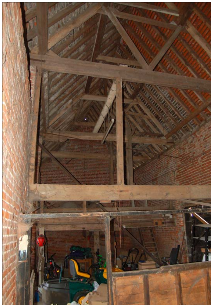
Plate 10 Victorian trusses viewed to north
