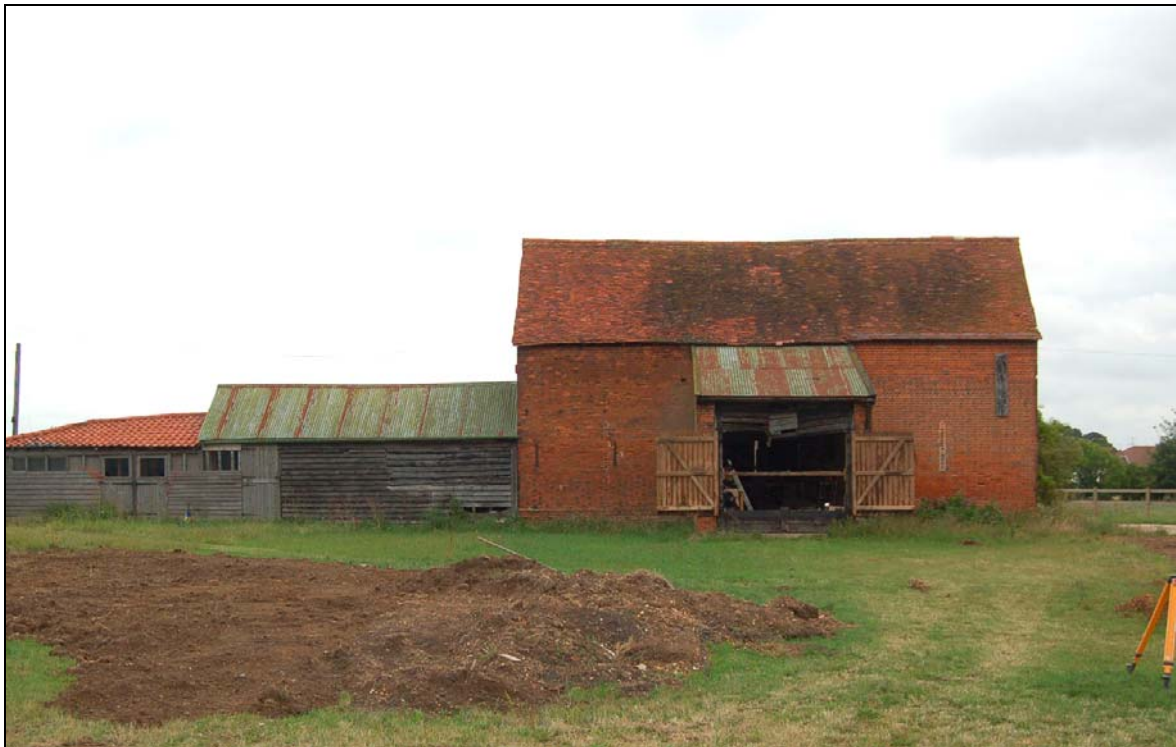
Plate 4 Barn 2 viewed to east
