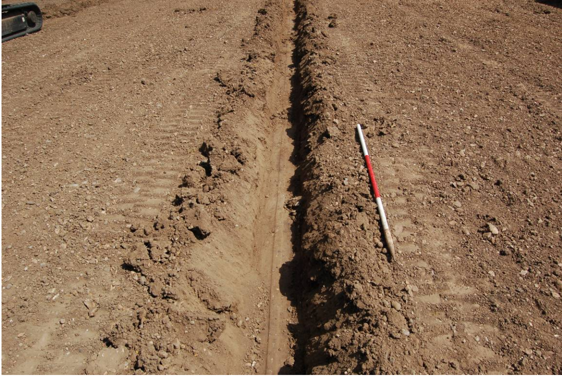
Plate 3: Detail showing location of Ditch 2 in drain run
