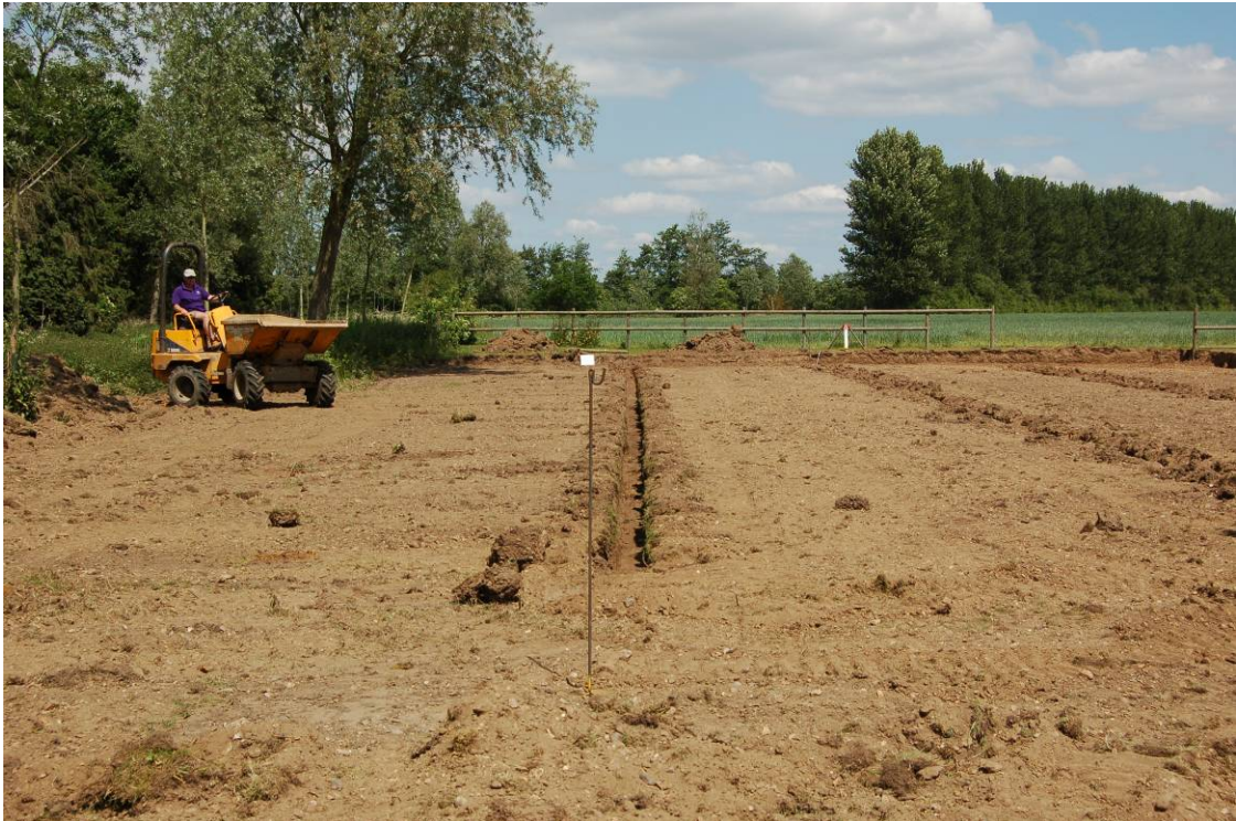
Plate 2: Drain runs (looking north)
