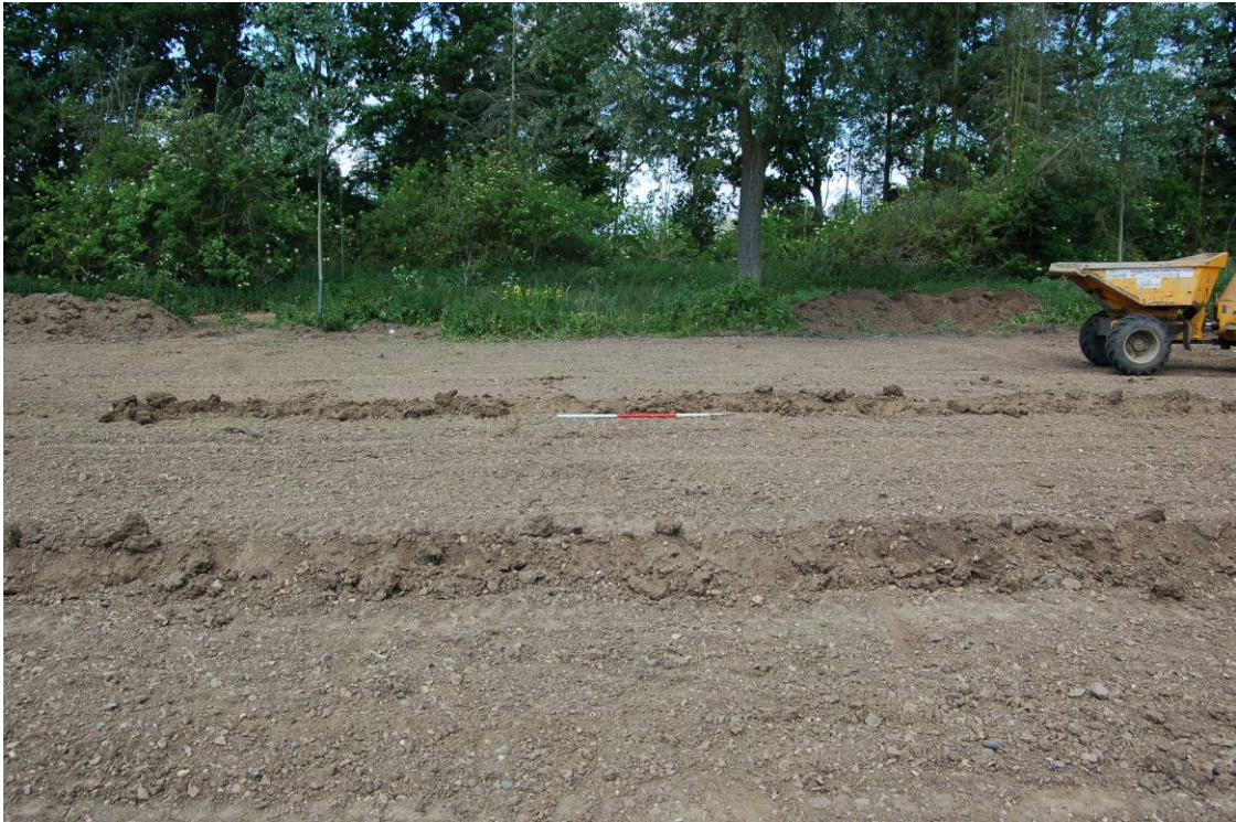
Plate 1: Arena following levelling and excavation of drain runs
