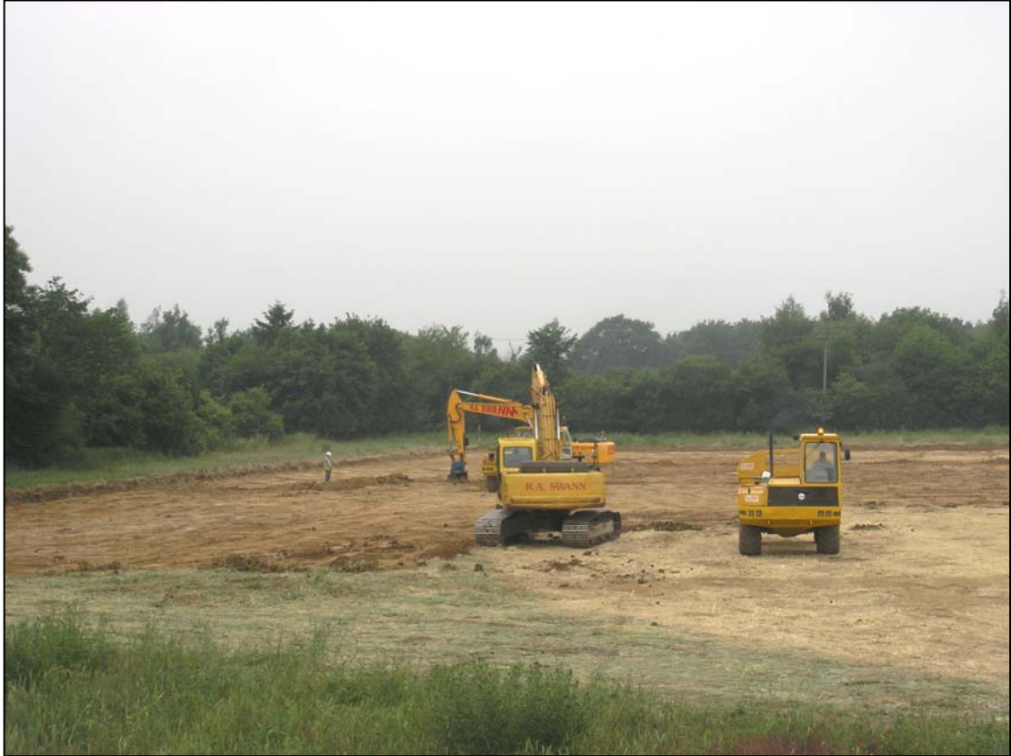
Plate 1: Topsoil and subsoil stripping Area 5
