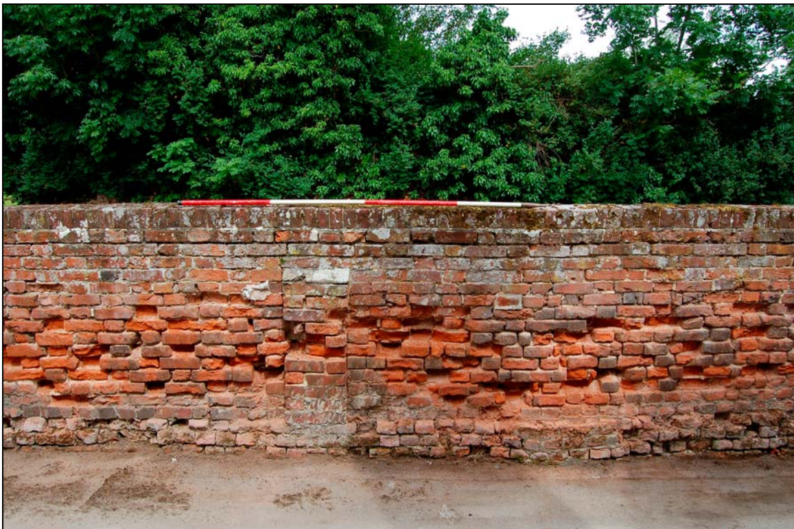
Plate 6 Historic phase 1 wall and central buttress below phase 2 rebuild (2m scale)
