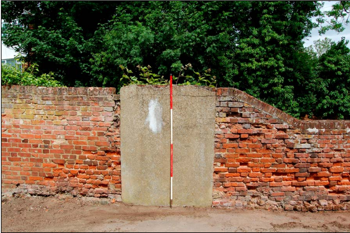
Plate 5 Evidence of phase 3 structure and modern wall across driveway (2m scale)
