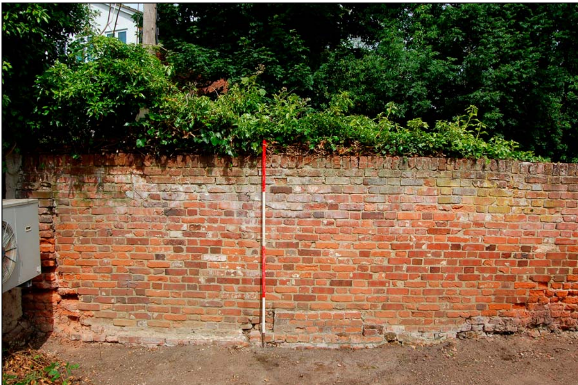
Plate 4 South-west historic buttress, pier base and modern phase 4 rebuild (2m scale)
