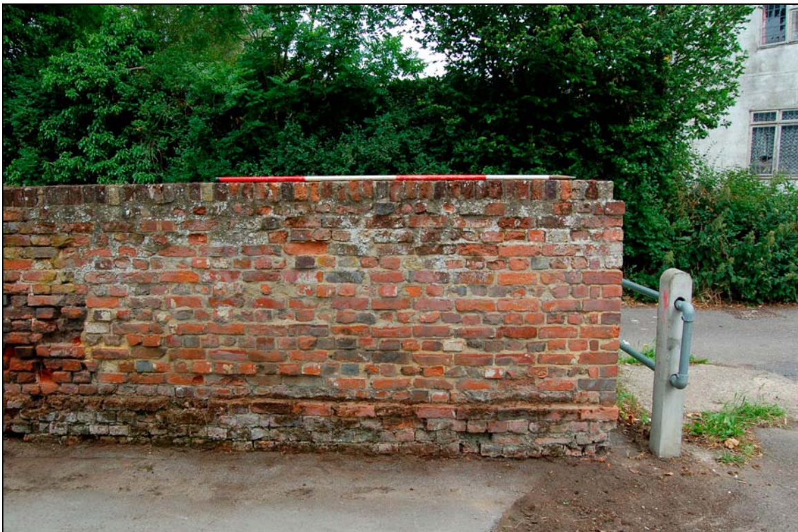
Plate 8 Phase 5 rebuild at north-east end (2m scale)
