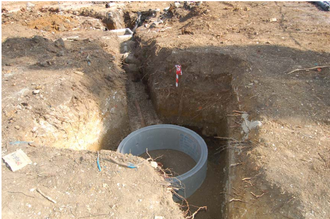
Plate 4: General view of sewer/ drain works
