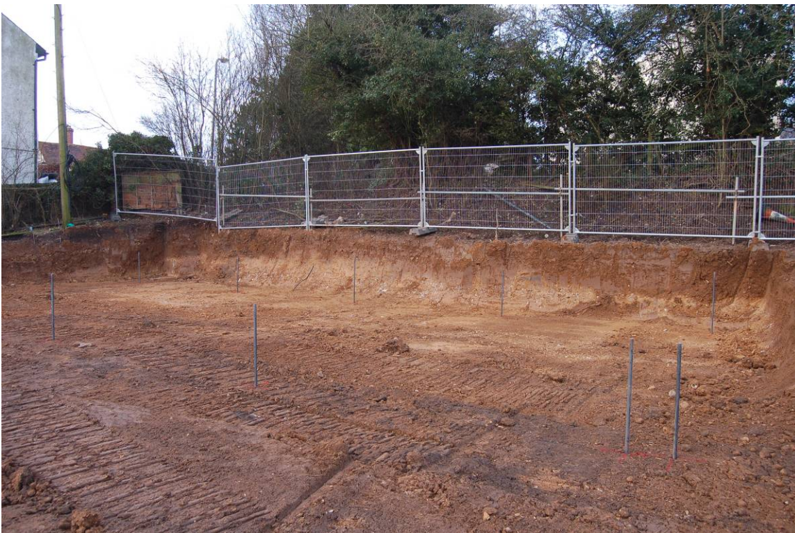
Plate 8: Plots 1 -3 and ground reduction at front of site
