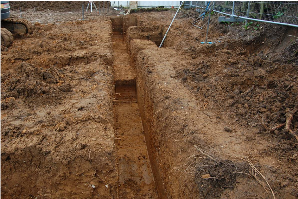
Plate 10: Plot 9 under excavation
