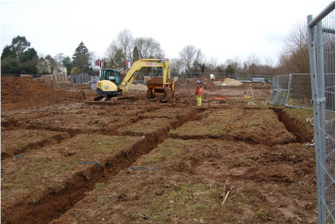
Plate 11: Plot 12 under excavation
