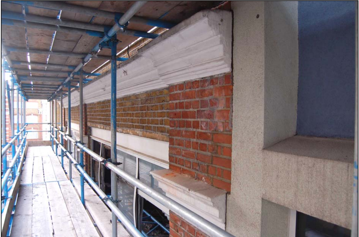
Plate 9 Cornice to original roofline
