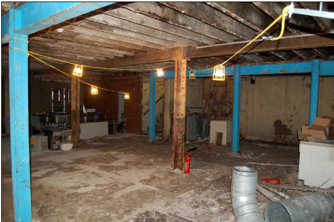
Plate 12 Basement under nos. 5-7 viewed to south-west
