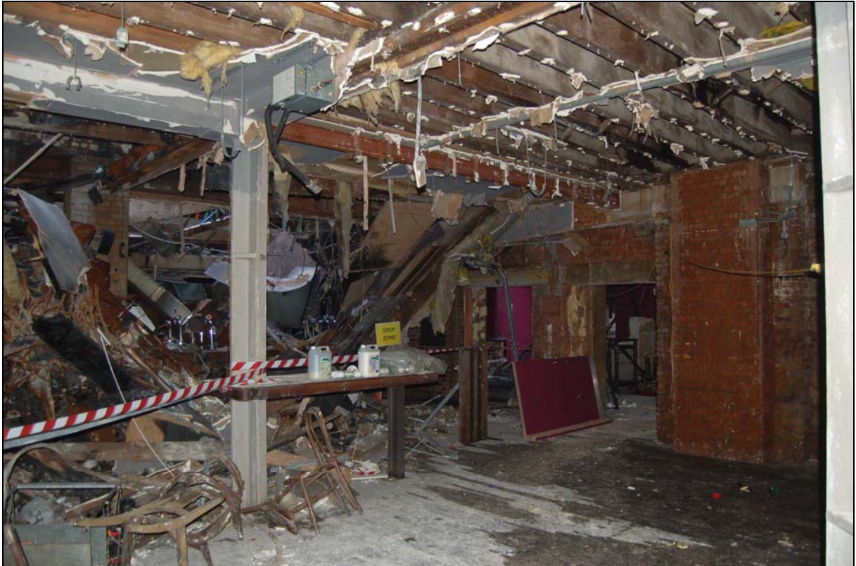
Plate 15 First floor of nos. 5-7 (bar) viewed to east (nos. 9-11)
