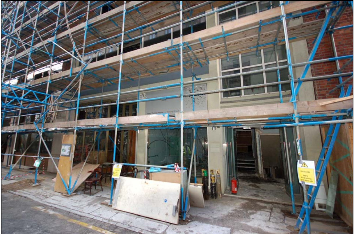
Plate 17 Ground floor frontage of nos. 9-11
