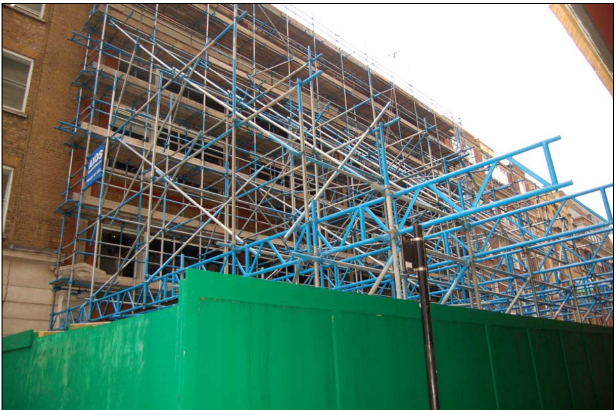
Plate 4 Scaffold across facade
