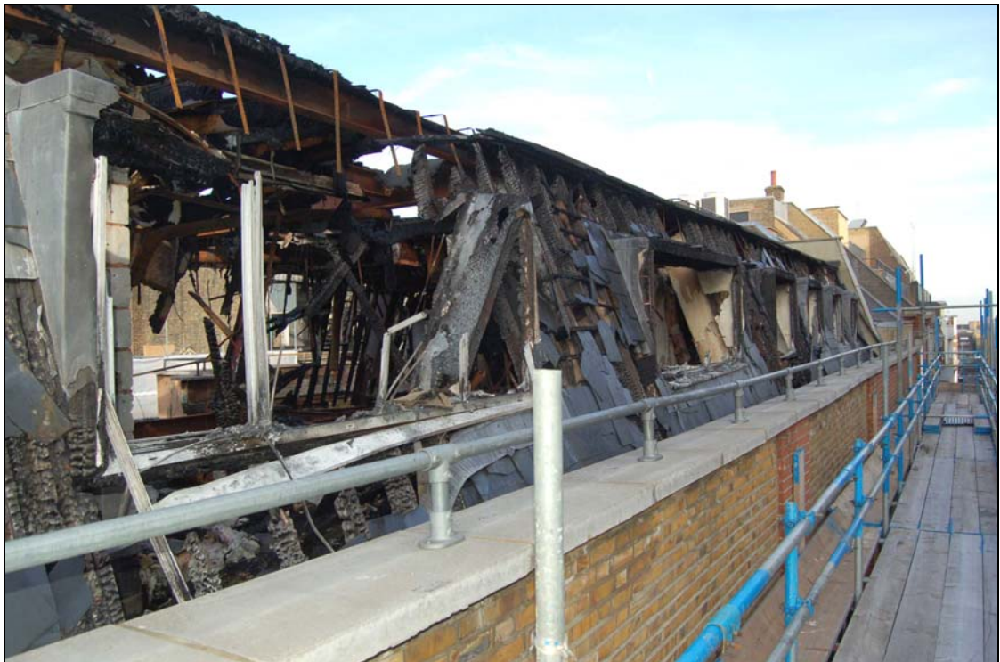
Plate 10 Modern roof viewed to east
