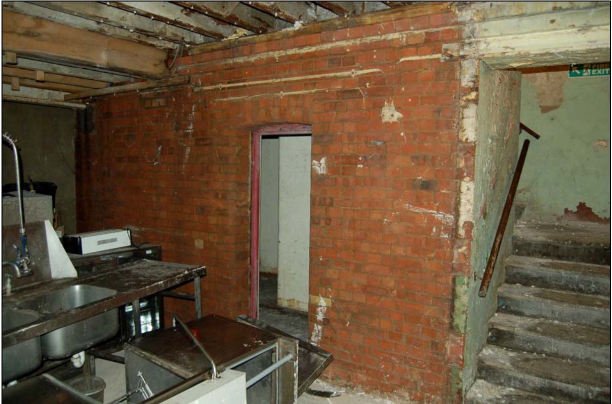
Plate 13 Storage area under stairs
