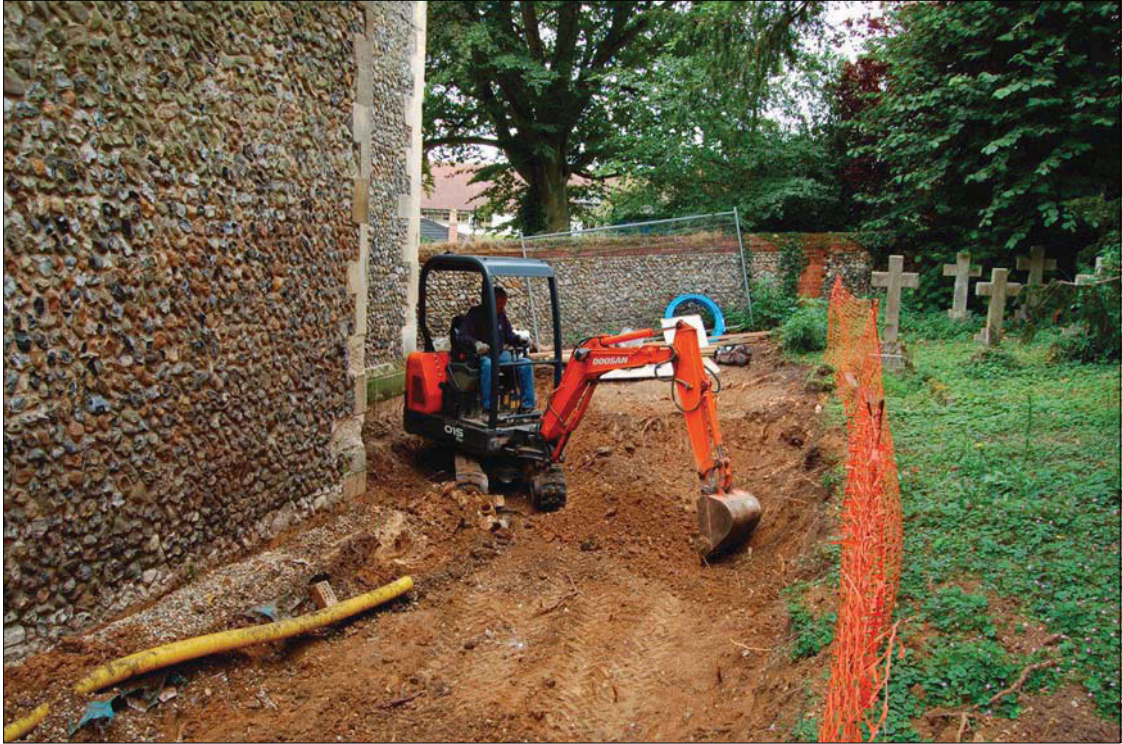
Plate 1. Extension footprint under excavation, looking west
