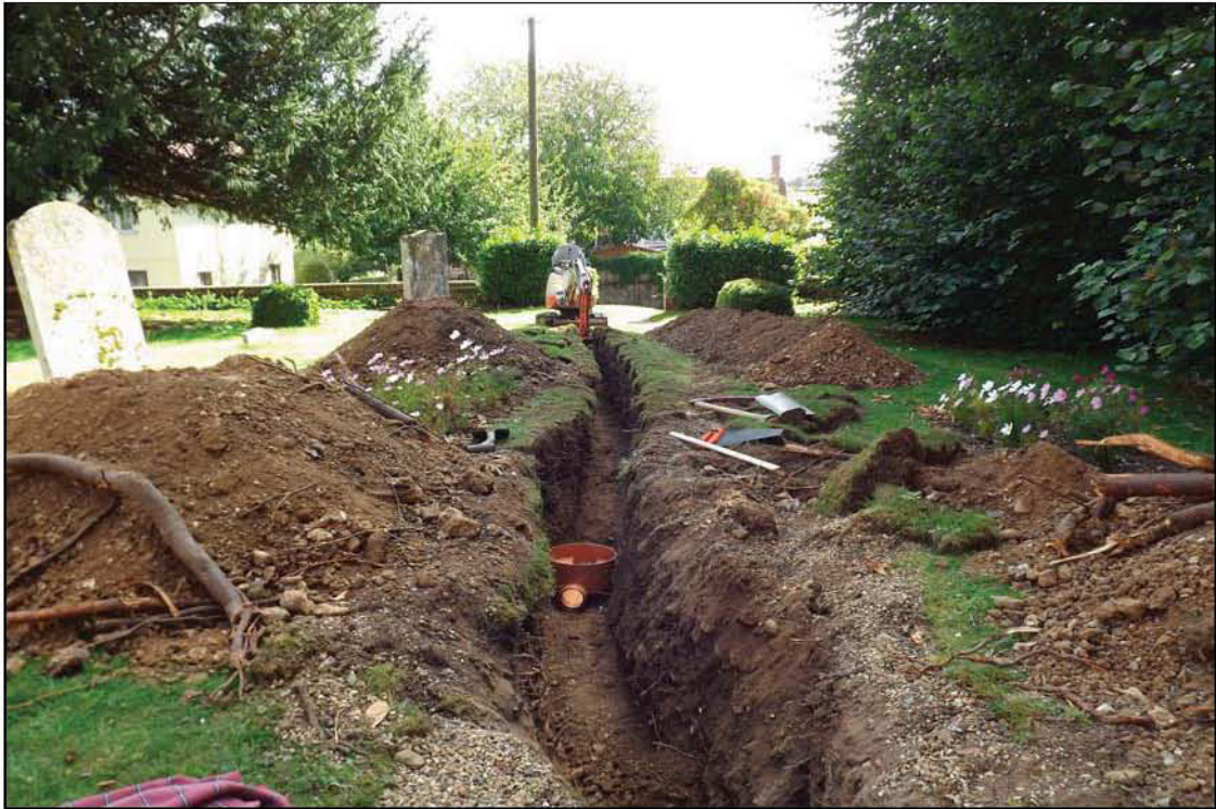
Plate 5. Drainage trench, looking south-east
